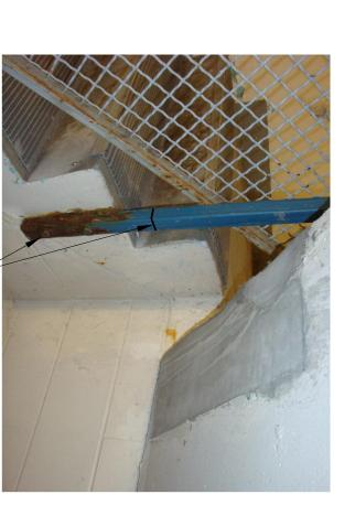
CUT OFF BOTTOM OF GUARDRAIL SUPPORT POST, WELD NEW SECTION TO POST TO REMAIN AND RE-ANCHOR TO STAIR RISER, BID ITEM #23
