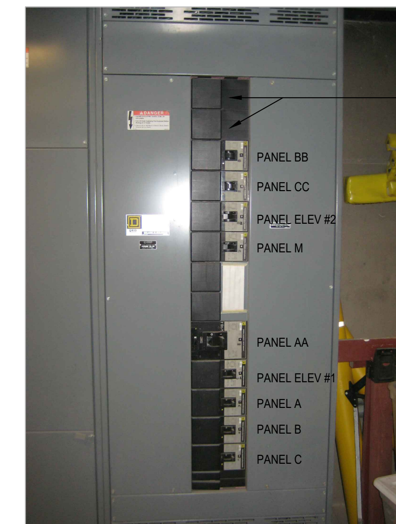
4 EXISTING SWITCHBOARD ELEVATION NO SCALE
