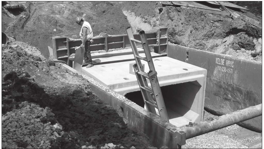
A new box culvert was added in Segment 1 to improve drainage in this low-lying area of the East Washington Avenue corridor between Blair Street and Thornton Avenue. Installing the box culvert among the many utility lines along the corridor was a challenging task.
