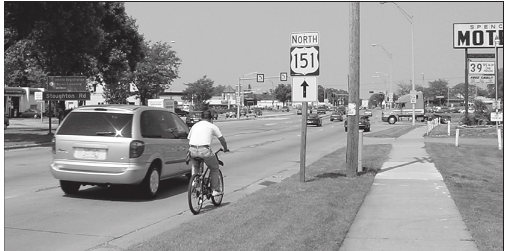
Construction on Segment 5 of the East Washington Avenue Reconstruction Project, from Melvin Court to Thierer Road, will start mid-March 2005.
