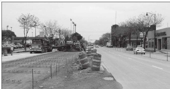
A new box culvert was added in Segment 1 to improve drainage in this low-lying area of the East Washington Avenue corridor between Blair Street and Thornton Avenue. Installing the box culvert among the many utility lines along the corridor was a challenging task.
