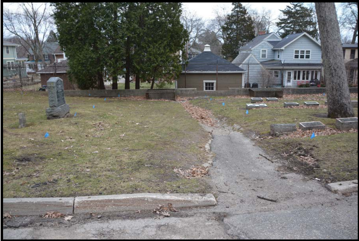
Figure Sixteen: Existing storm sewer to be refurbished.
