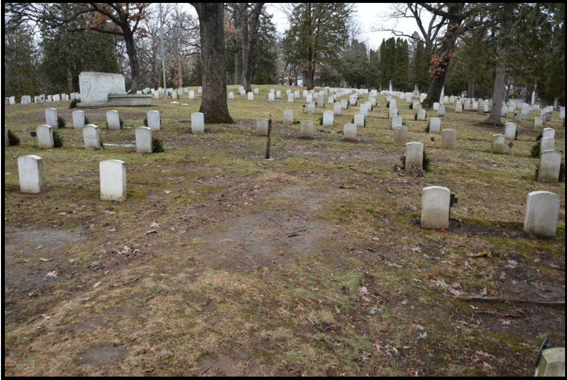
Figure Six: Existing standpipe (center of image) to be removed at DA-134.
