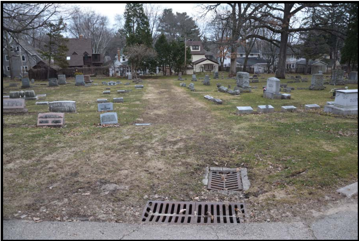
Figure Seventeen: Existing storm sewer to be refurbished.
