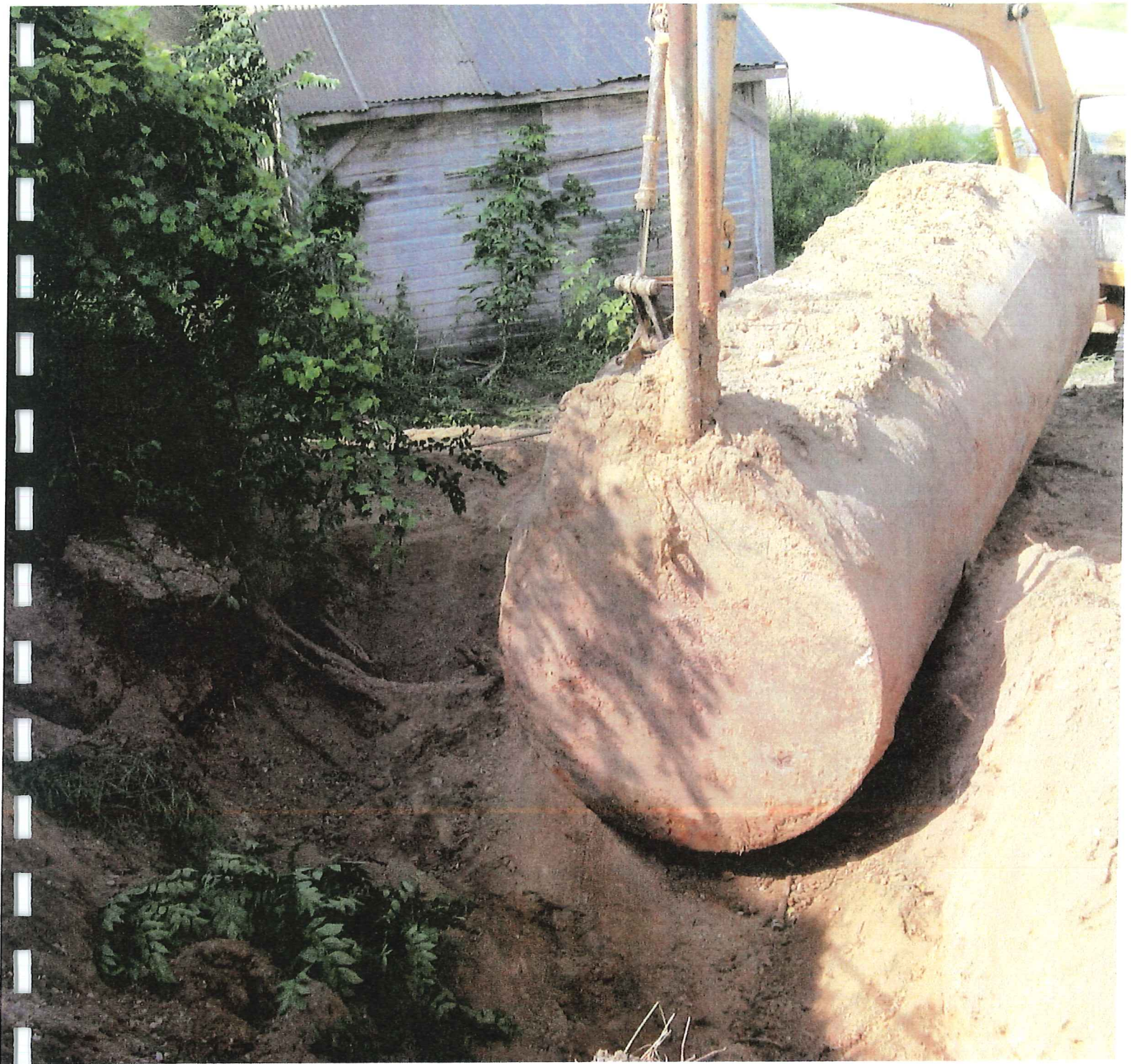
PHOTO 2: UST AFTER REMOVAL
