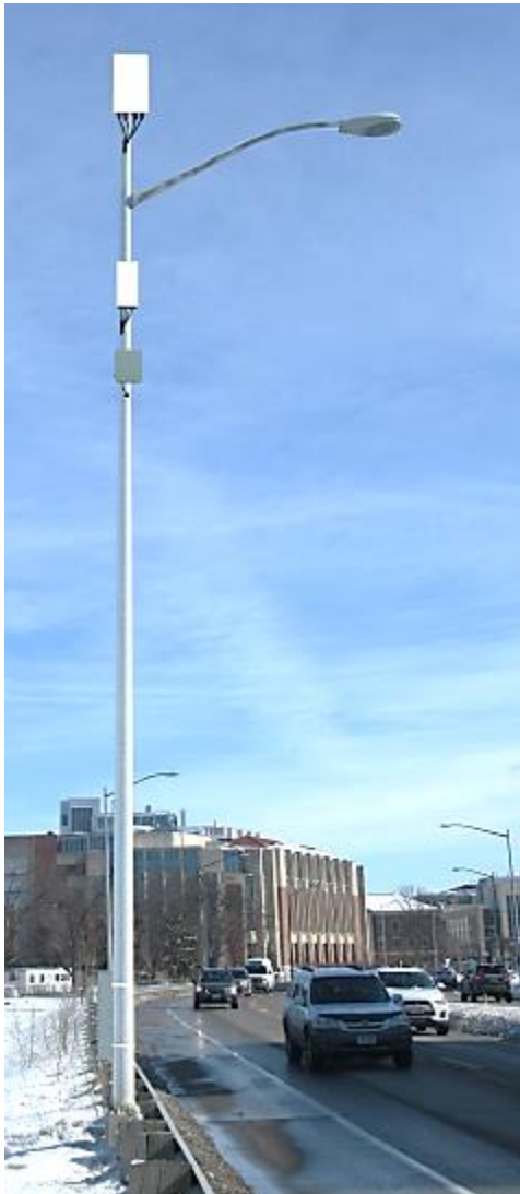
Figure 8-6: Collocated Small Cell Example using a different technology; not an approved design
