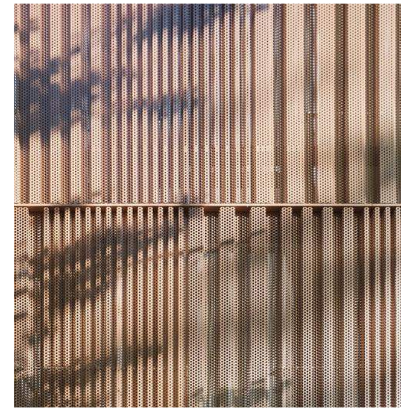
Perforated Metal Panel (@ Parking)
