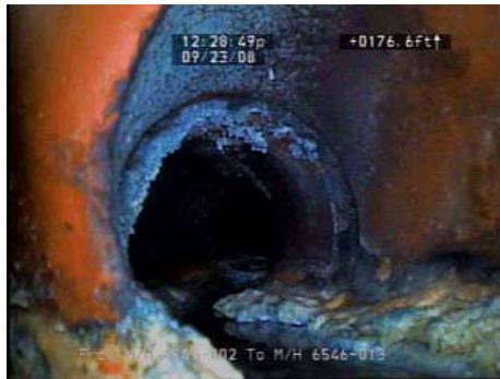
Private sewer lateral and City's sewer main affected by FOG
