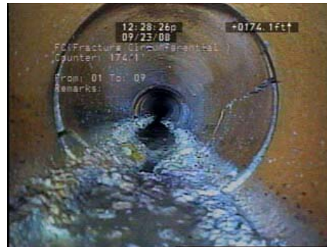
Private sewer lateral and City's sewer main affected by FOG
