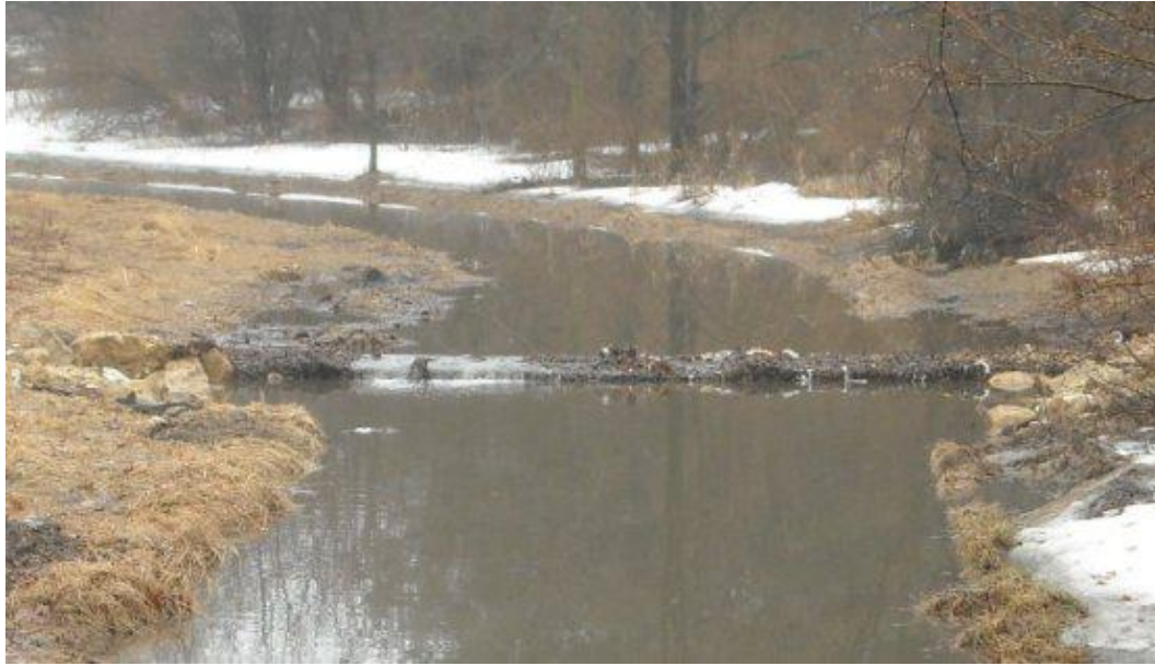
Warner Park Gabion
