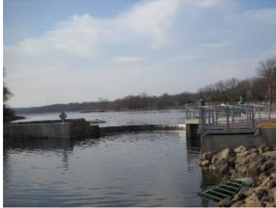
Wingra Dam, after
