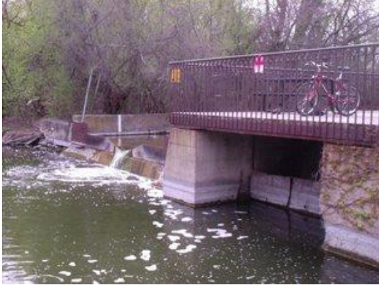
Wingra Dam, before
