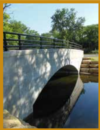
Tenney Park Bridge
