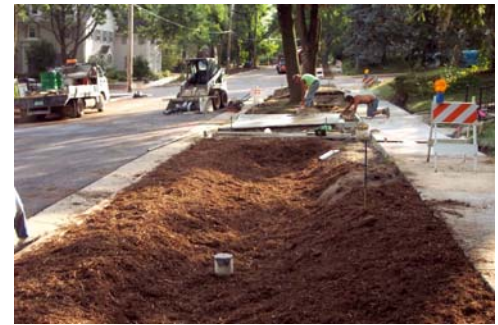
Adams Street rain garden installation.
