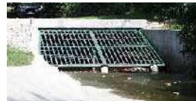
Storm water culvert
