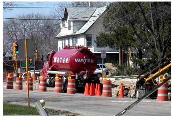
Water distribution system pipe replacement on First Street.
