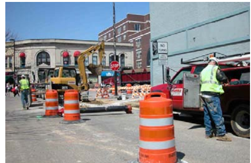
Replacement of sanitary sewer mains along Broom Street.
