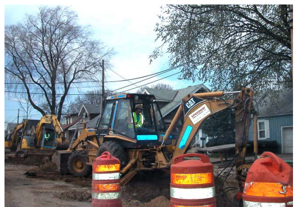
Utility replacement on First Street.
