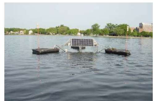
SolarBees are solar powered water circulators being tested as a means of monitoring and controlling blue-green algae blooms in Monona Bay.
