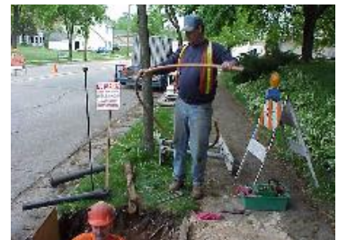
Lead pipe replacement.
