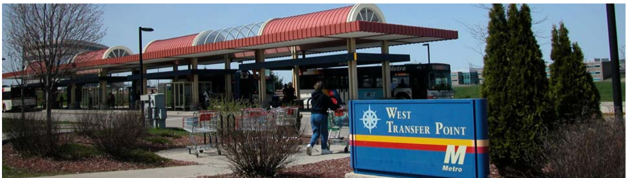
Metro Transit West Transfer Point
