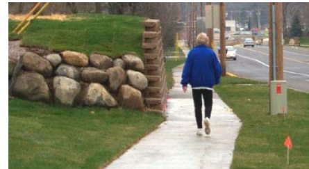
New sidewalk along Buckeye Road.
