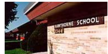
Hawthorne Elementary School
