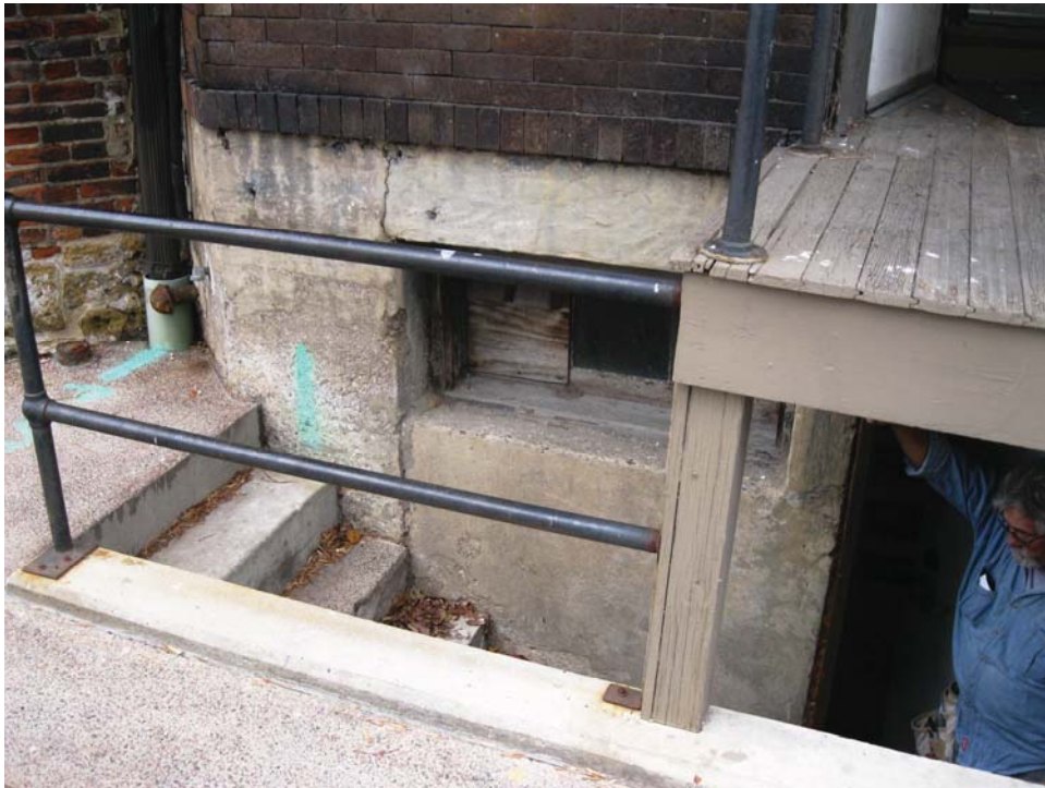
Photo 4 – Stair to basement from Fairchild Street
