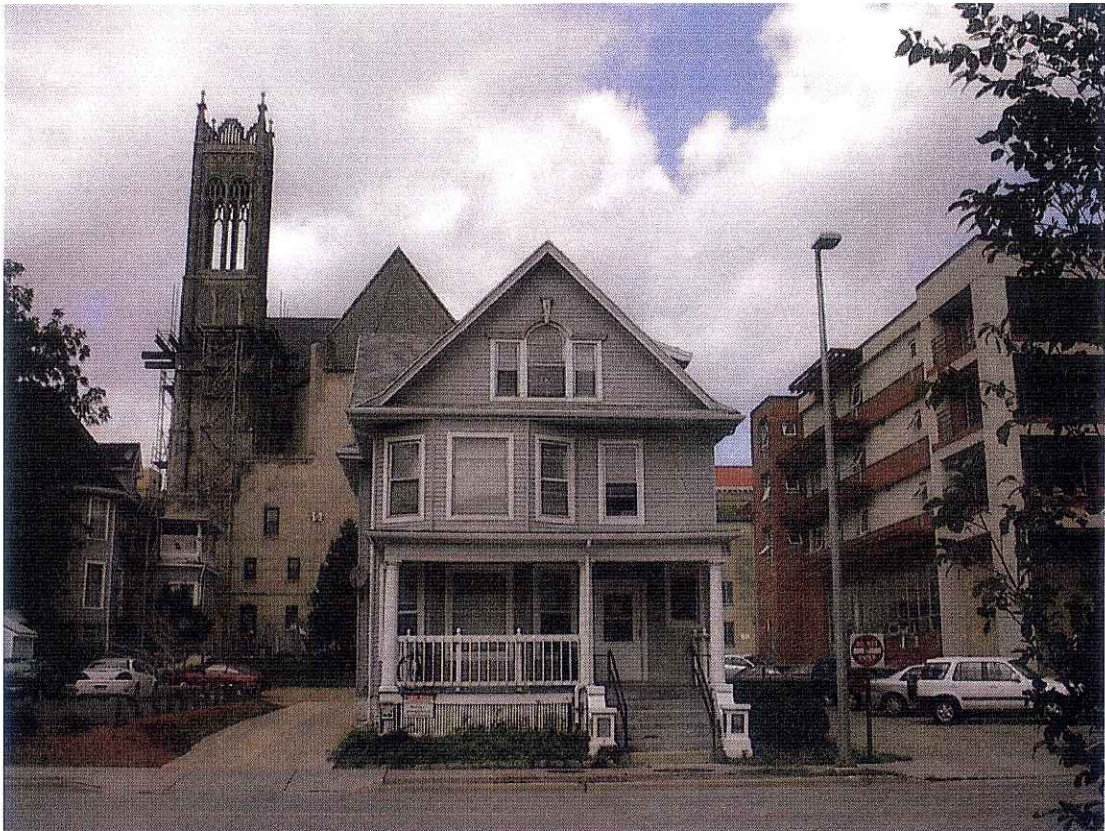
1. 1022 W. Johnson Street - Front
