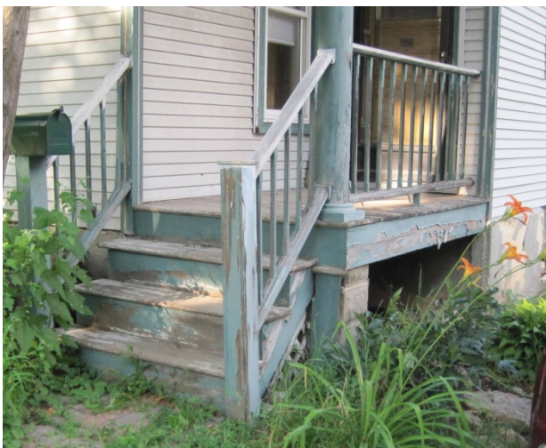
315 S. Mills St. CONDITION EXAMPLES FRONT PORCH
