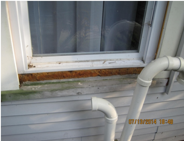
315 S. Mills St. CONDITION EXAMPLES IMPROPERLY SIZED WINDOW - NORTH SIDE
