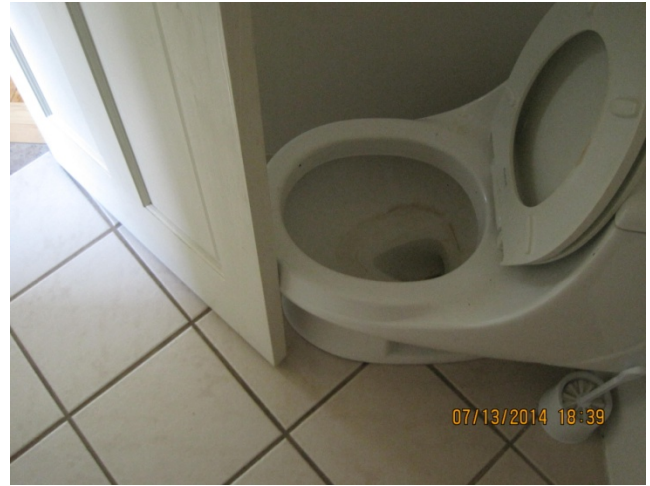
315 S. Mills St. CONDITION EXAMPLES MAIN BATHROOM
