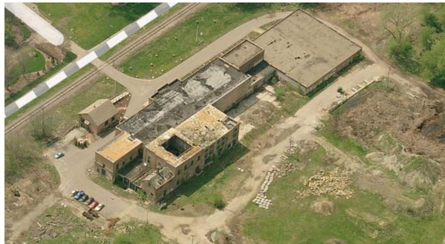
EXISTING NORTH FACADE AERIAL
