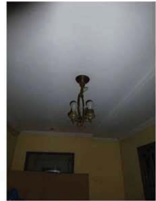
Image 10 Original light fixture, main entry, first floor
