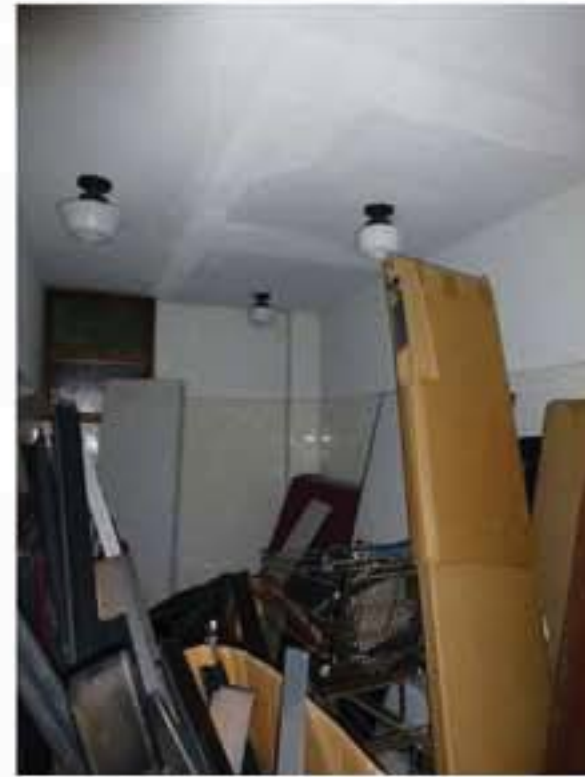
Image 7 Restroom with original light fixtures
