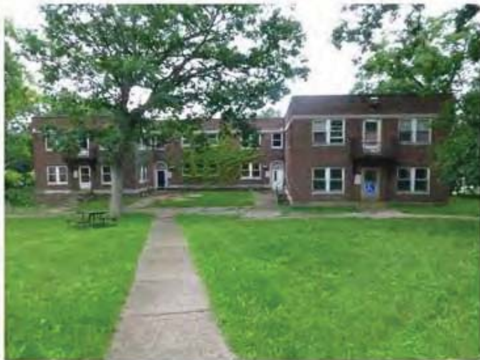
Image 3 Dormitory for Help - view from the top of the hill to existing courtyard
