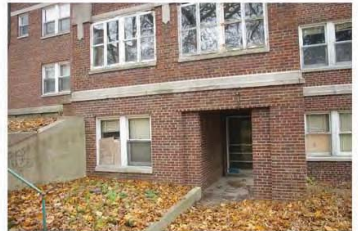
Image 5 Dormitory for Help - exterior wall to be retained below water table and window opening infilled with salvaged and interactive materials.
