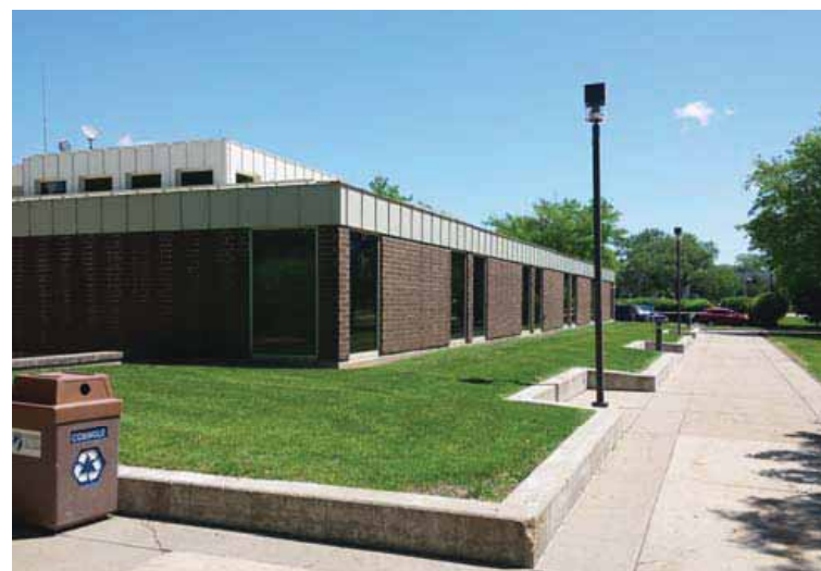
ADMINISTRATIVE BUILDING - SOUTH FACE
