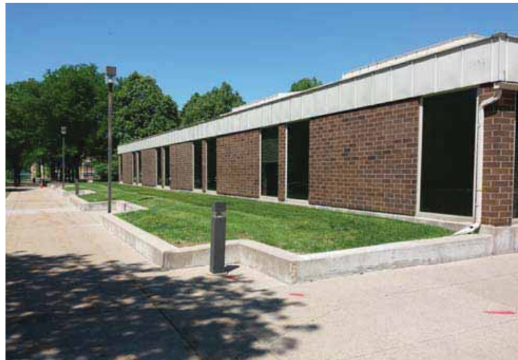
ADMINISTRATIVE BUILDING - SOUTH FACE
