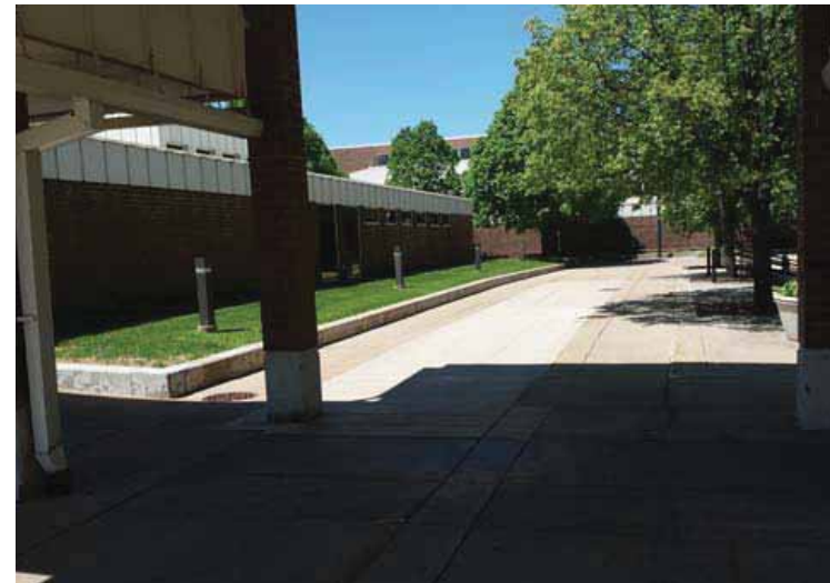
ADMINISTRATIVE BUILDING - NORTH FACE
