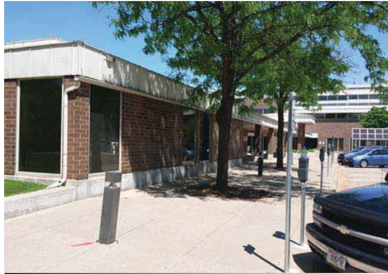
ADMINISTRATIVE BUILDING - EAST FACE
