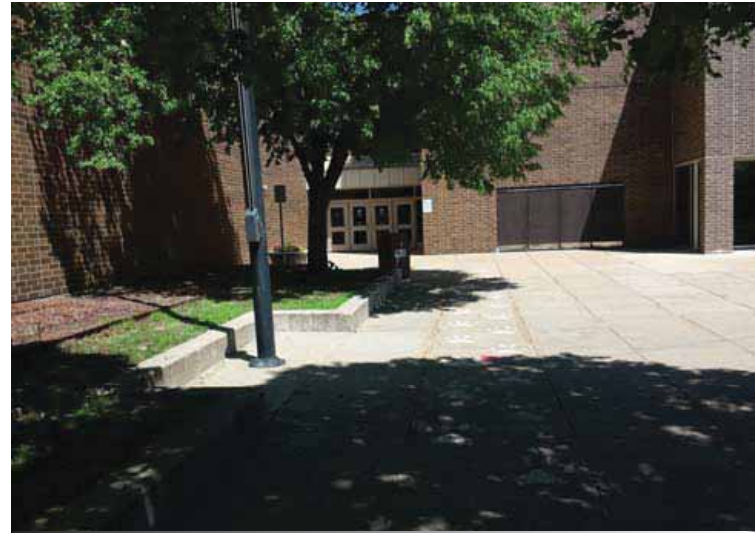
ENTRANCE TO GYMNASIUM STAIRWELL
