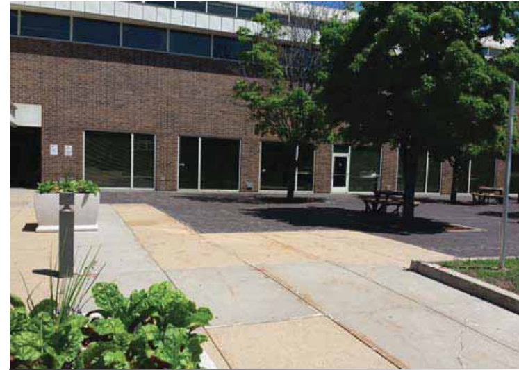
VIEW NORTH INTO MAIN PLAZA
