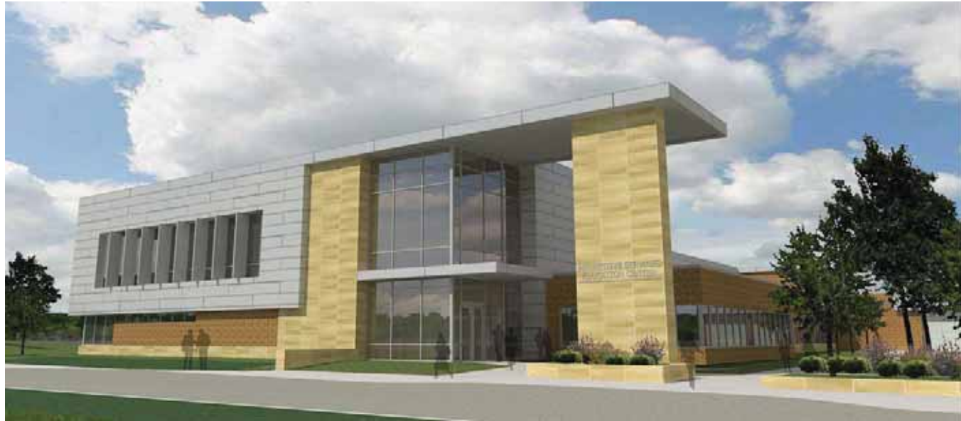
Northeast Ground View
