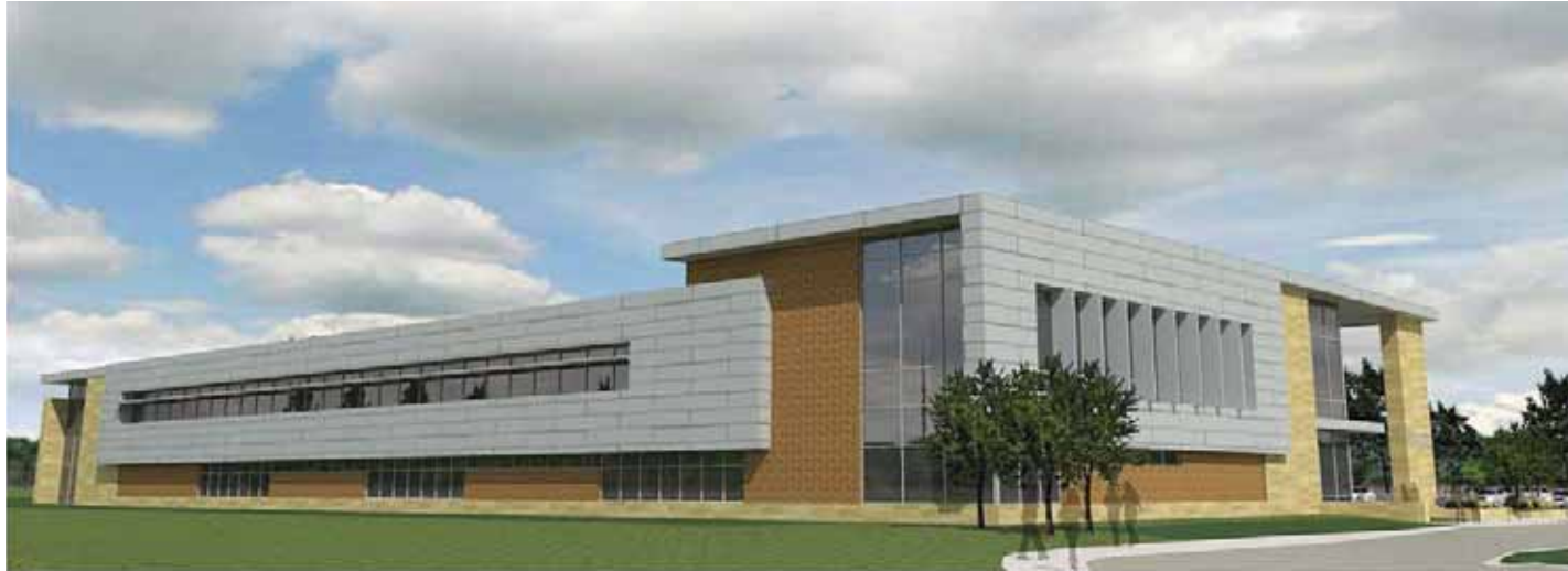
Southeast Ground View
