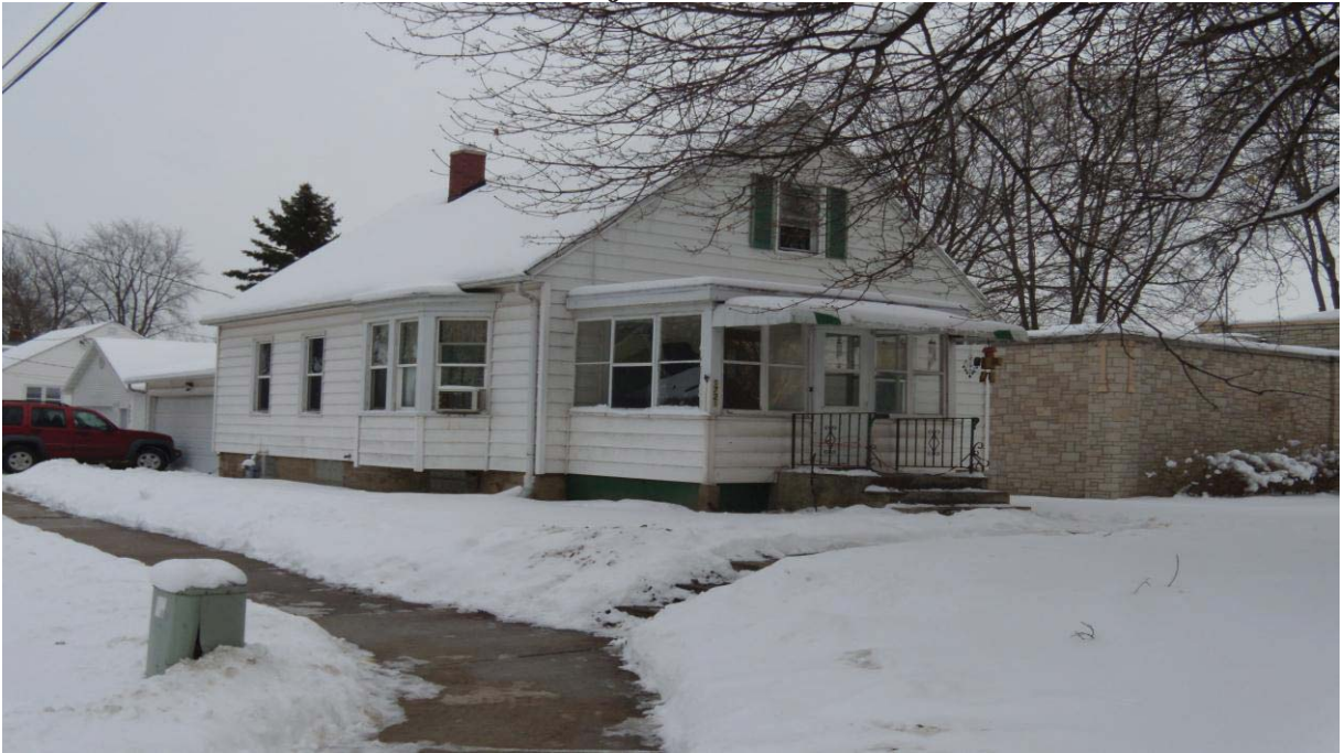
Subject. View Toward SE from NW.
