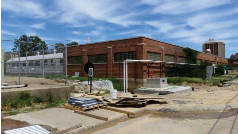
View 11: Southwest corner of building (current utility work in progress)
