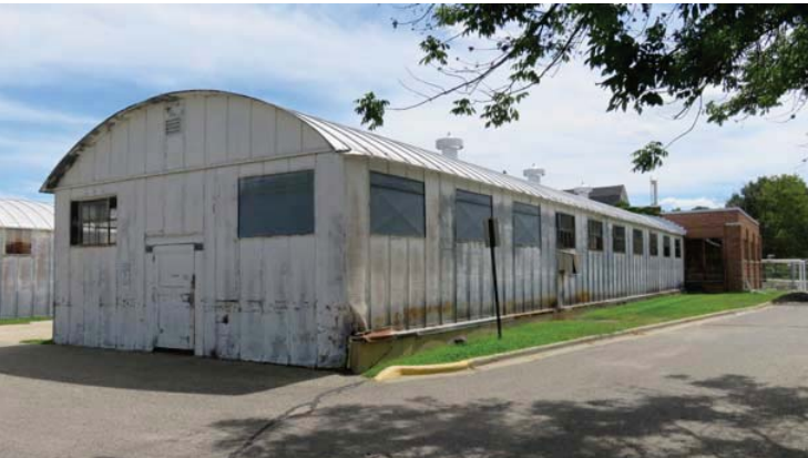
View 9: Northwest corner of building
