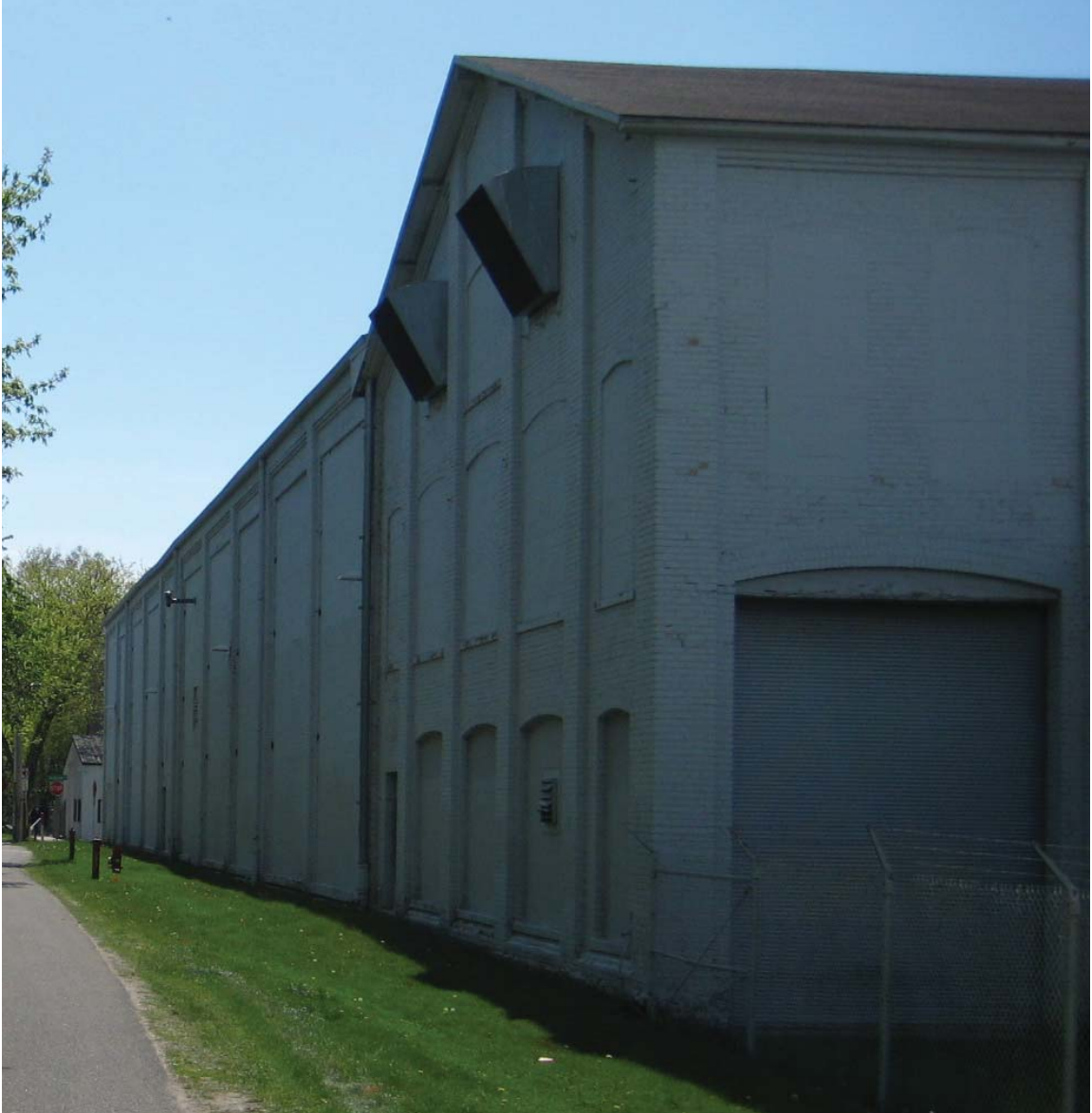
Photo #8 - Site photo looking southwest
