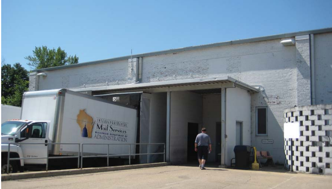
Photo #27 - Site photo looking southwest
