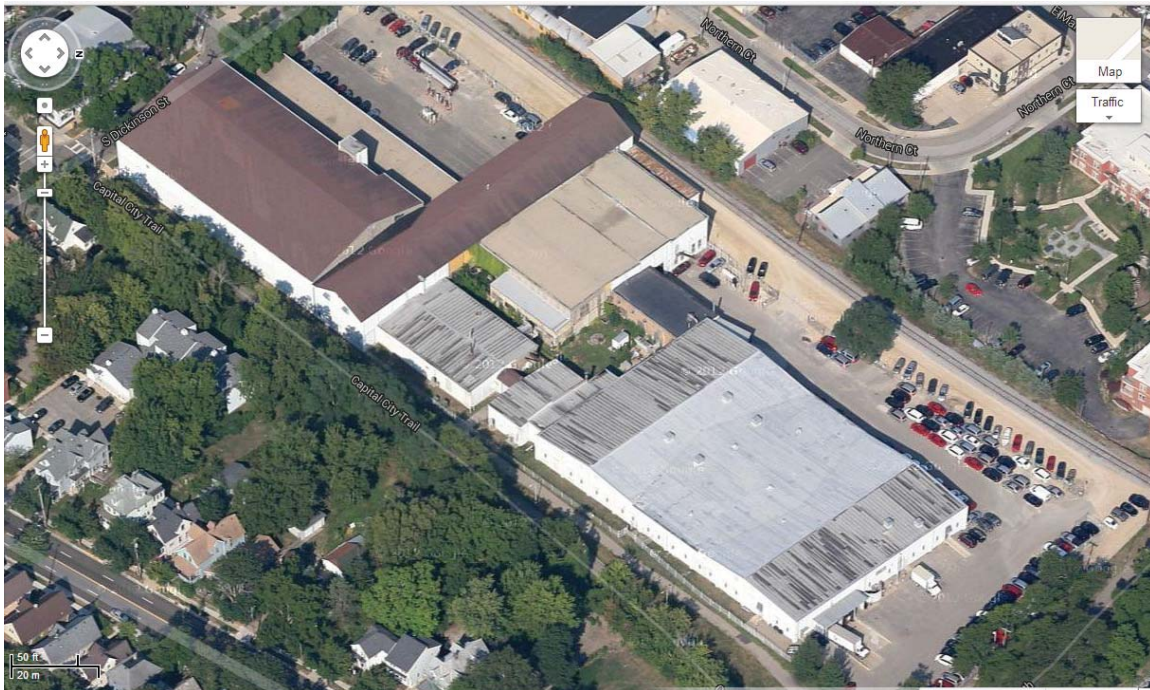
Photo C - Aerial view looking west
