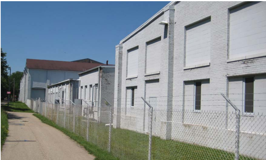
Photo #6 - Site photo looking southwest
