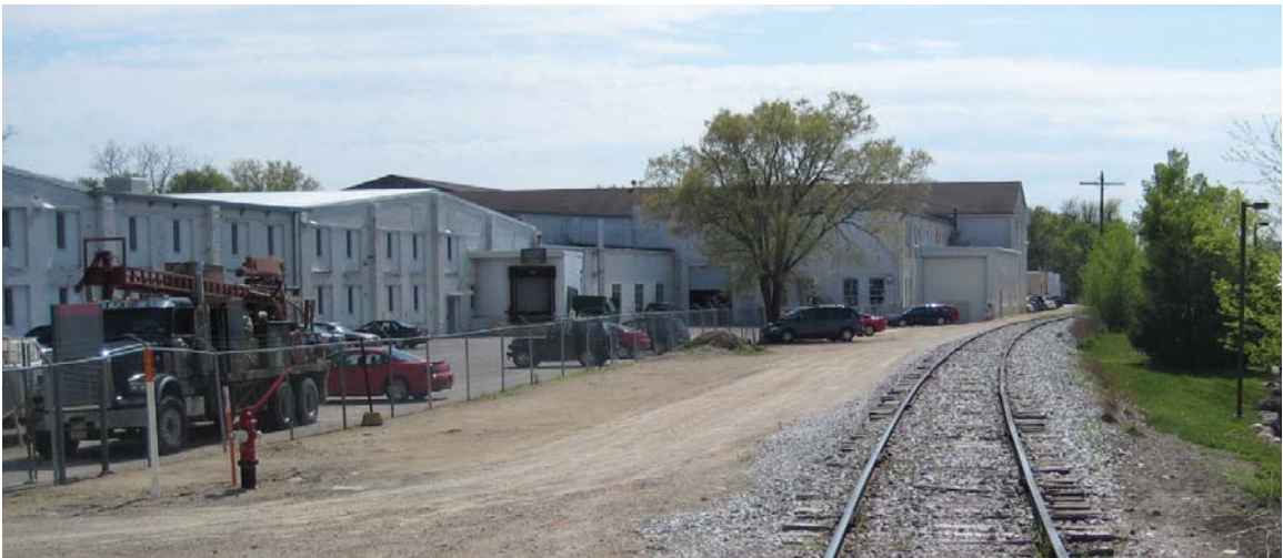
Photo #22 - Site photo looking southwest
