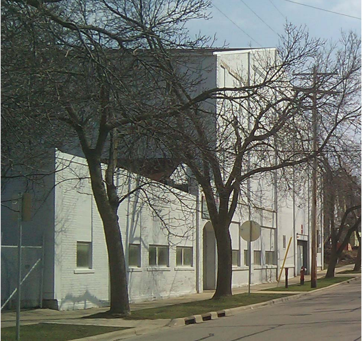
Photo #12 - Site photo looking east
