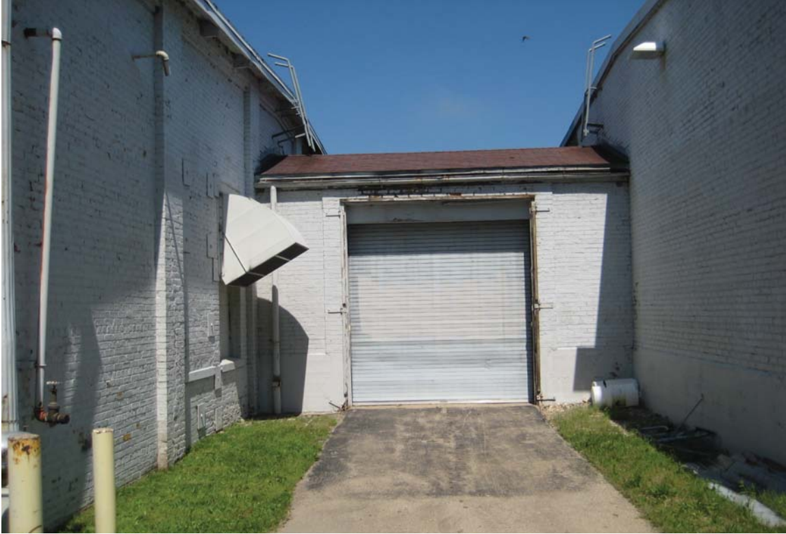
Photo #7 - Site photo looking northwest
