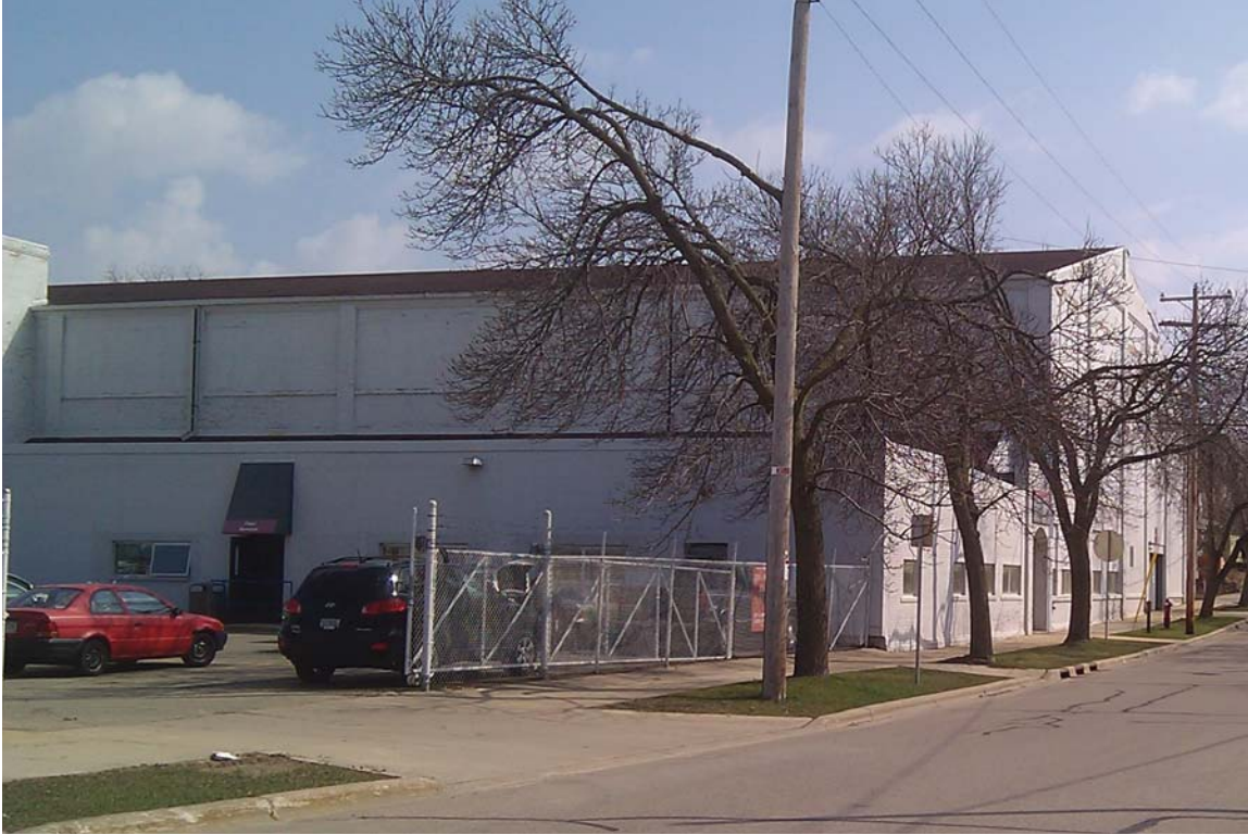
Photo #13 - Site photo looking east
