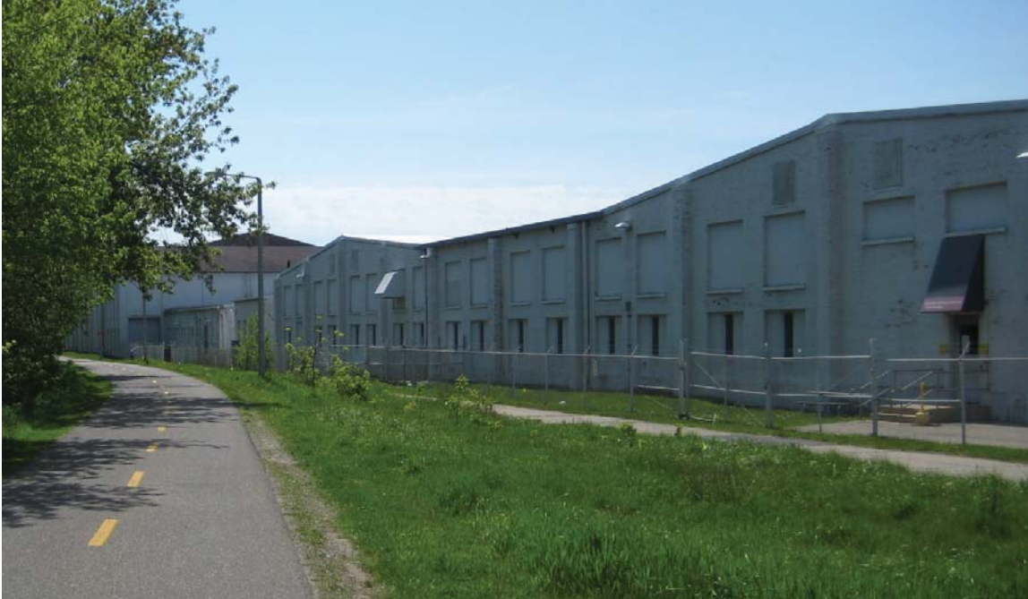
Photo #3 - Site photo looking southwest
