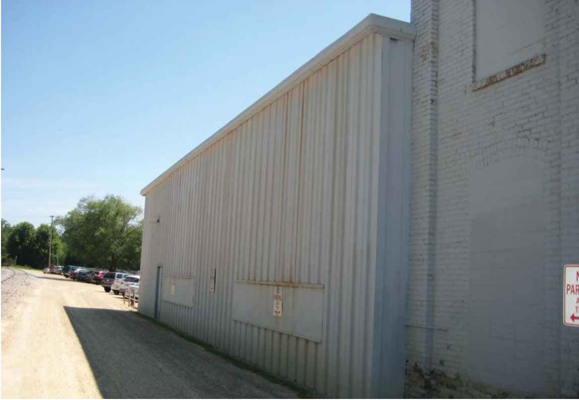
Photo #19 - Site photo looking east
