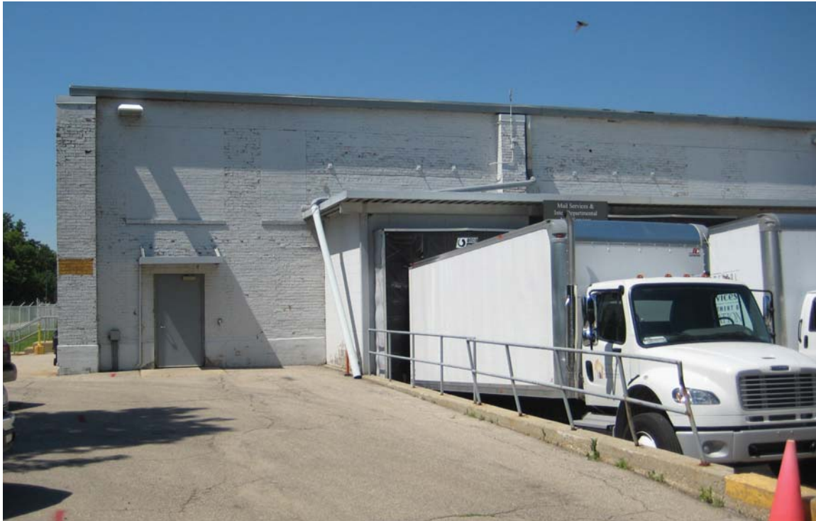
Photo #28 - Site photo looking southwest
