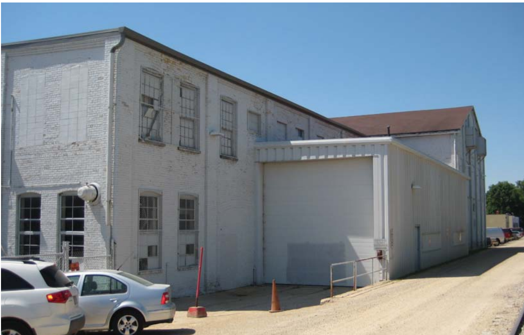
Photo #20 - Site photo looking southwest
