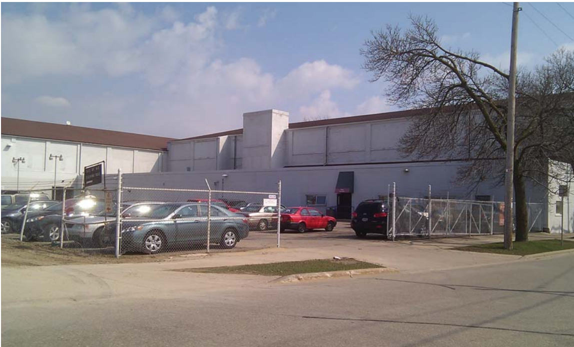
Photo #14 - Site photo looking east
