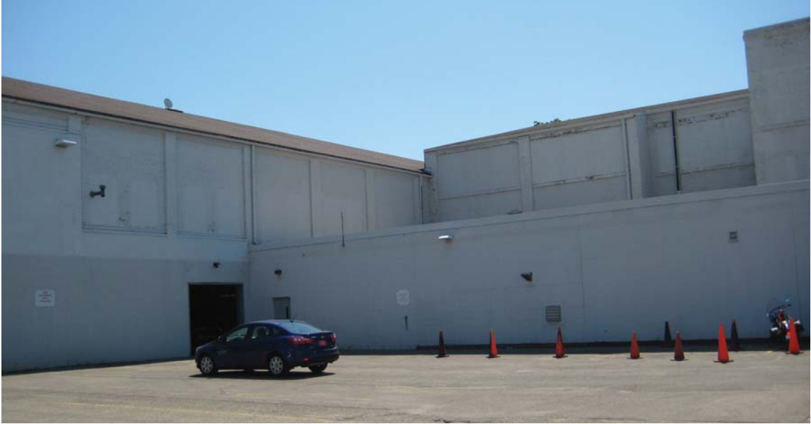
Photo #15 - Site photo looking east
