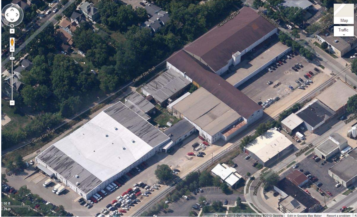
Photo B - Aerial view looking south
