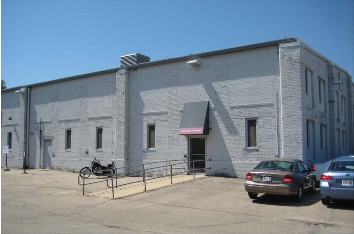
Photo #25 - Site photo looking southwest
