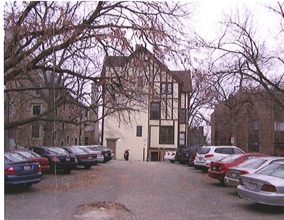
210 Langdon Street - Rear Elevation
