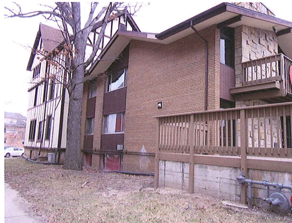
210 Langdon Street - Side Elevation
