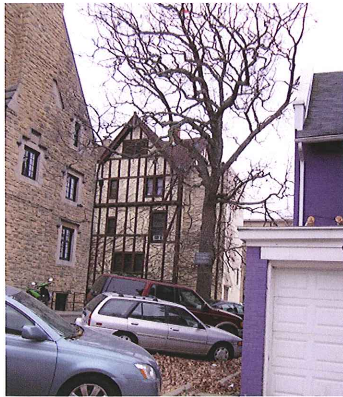
210 Langdon Street - Side Elevation
