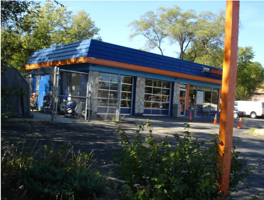
NE Corner of Site to Building
