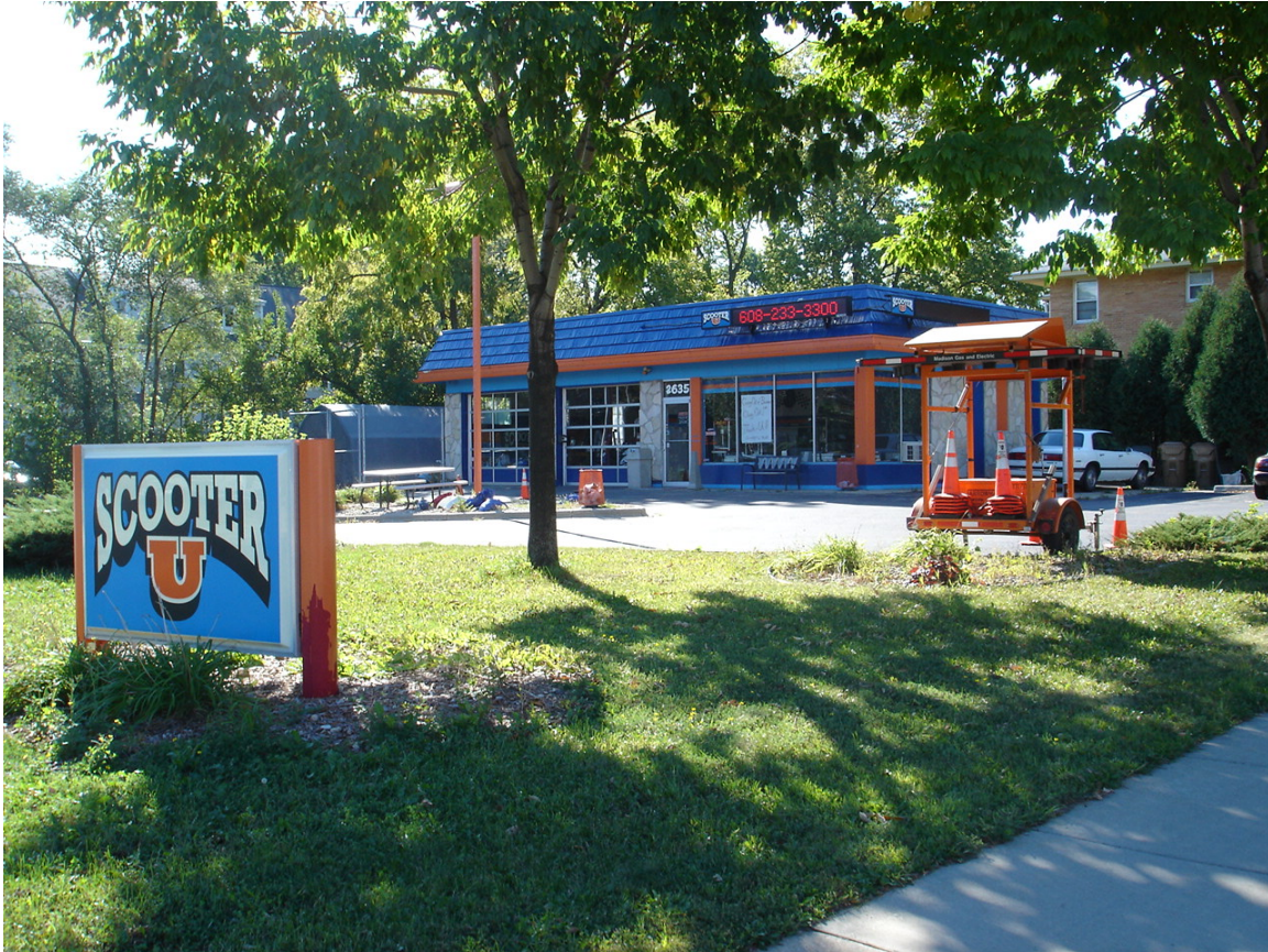
NW Corner of Site to Building
