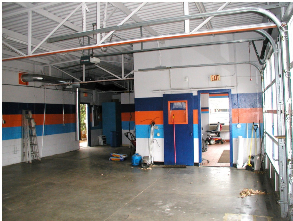
Shop Area Interior of Building
