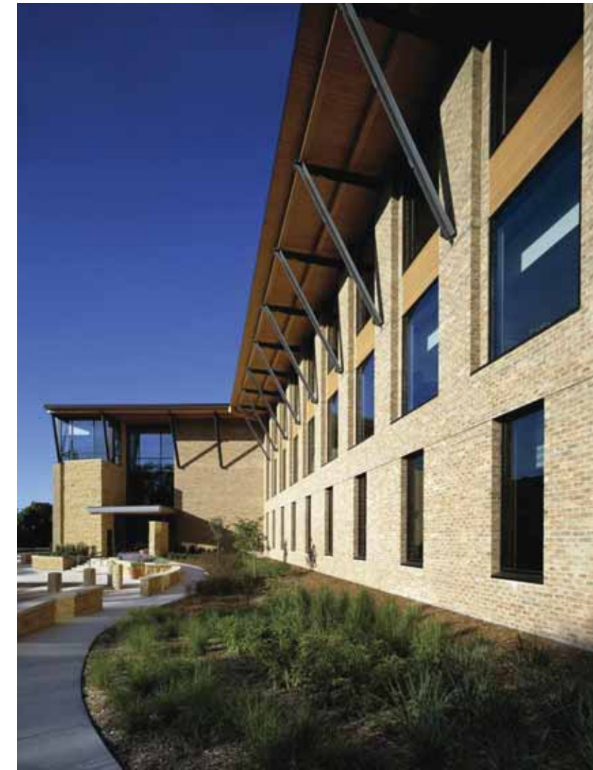
View of Existing Findorff Building - Parking Lot Landscaping and Existing Entry
