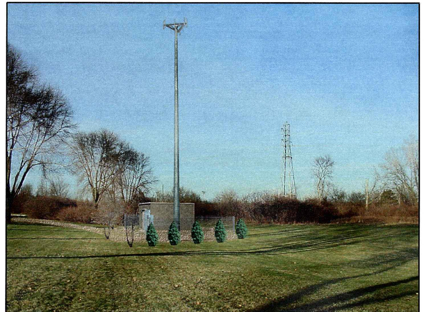
LOOKING NORTH AT PROPOSED US CELLULAR COMPOUND & MONOPOLE
