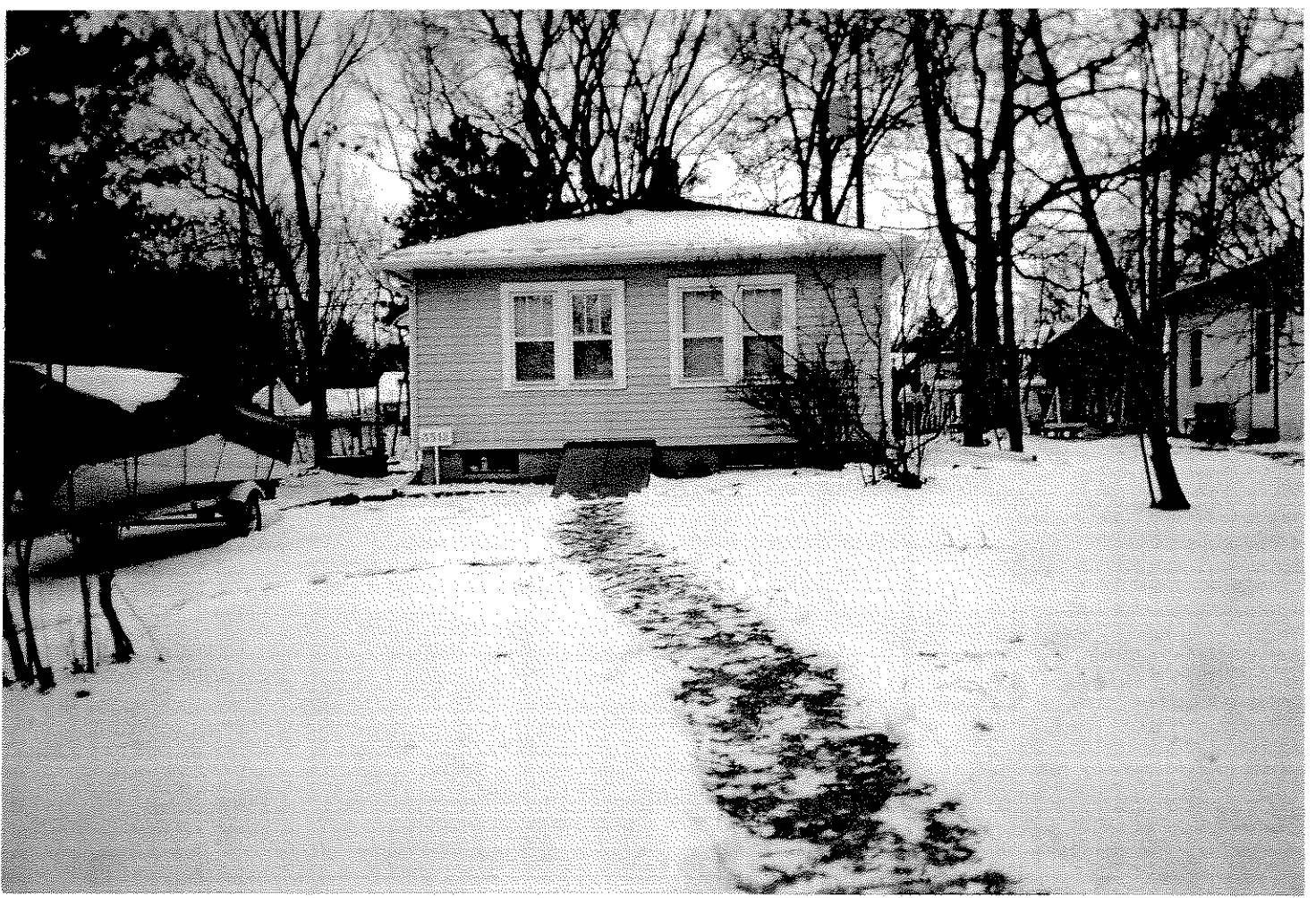
Existing house at 3512 Gregory St. to be demolished.
