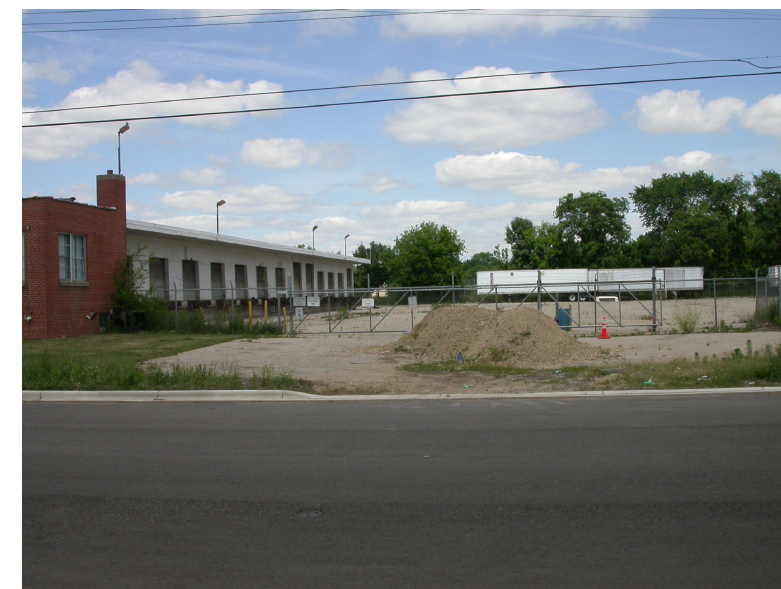
VIEW FROM N. THIRD STREET LOOKING NORTHEAST
