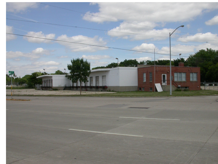
VIEW FROM PENNSYLVANIA AVENUE AND THIRD STREET LOOKING NORTHEAST
