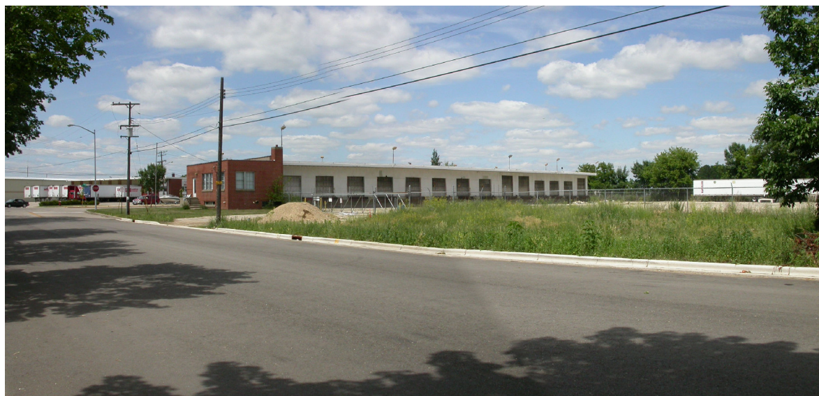
VIEW FROM N. THIRD STREET LOOKING NORTH
