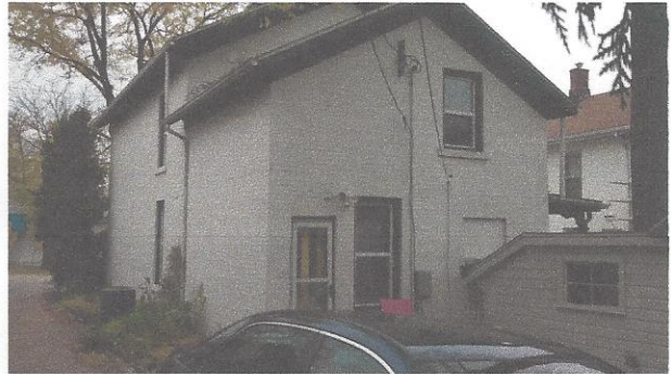
View of Rear
