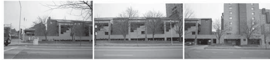
5 EXISTING STREETScape AT OPPOSITE SIDE OF BROOM STREET
