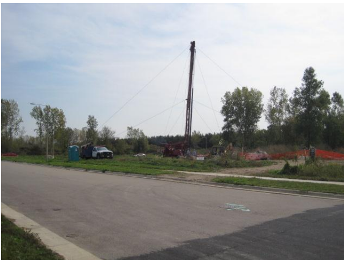
Project site - viewed from northwest
