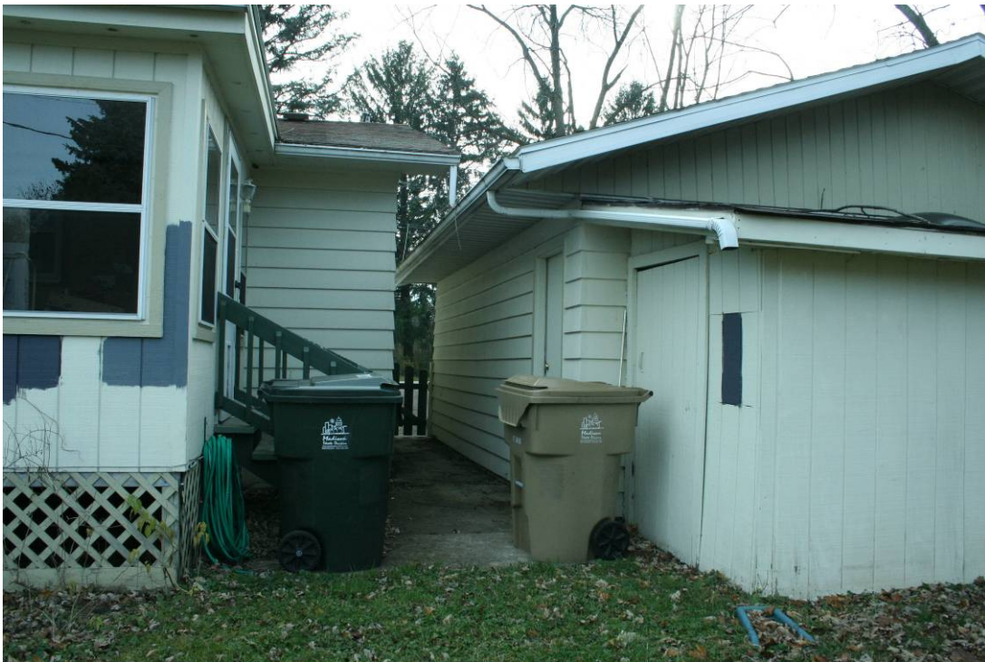
4908 Three season porch and garage (rear of building) Lean-to shed is in need of re-building
