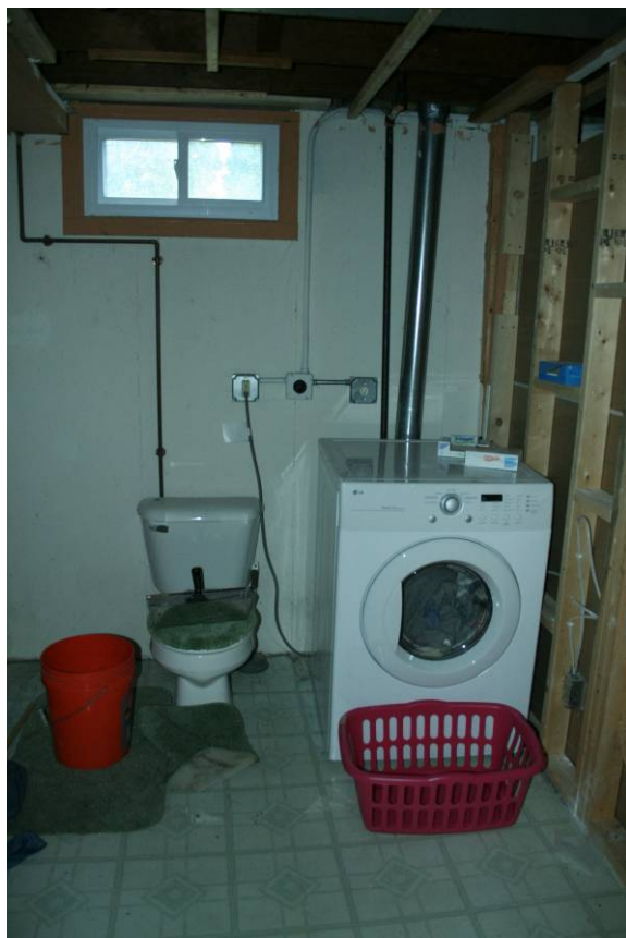
4908 Basement bath and Laundry
