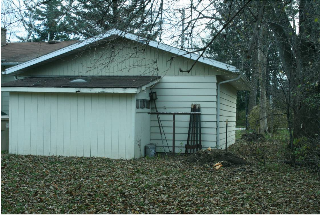
4908 Back of garage
