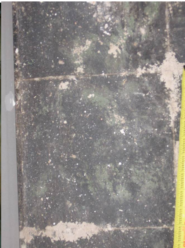
4908 Asbestos tile floor
