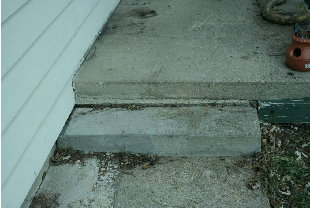
4908 Entrance steps and sidewalk – replacement is recommended
