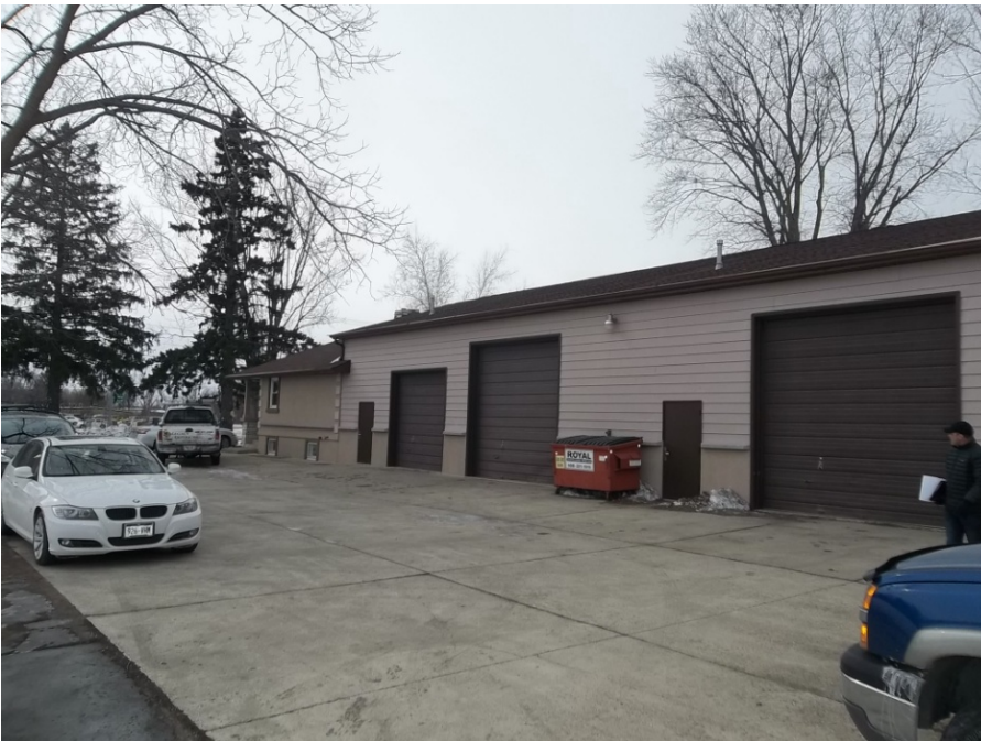
NE Site to the Building
