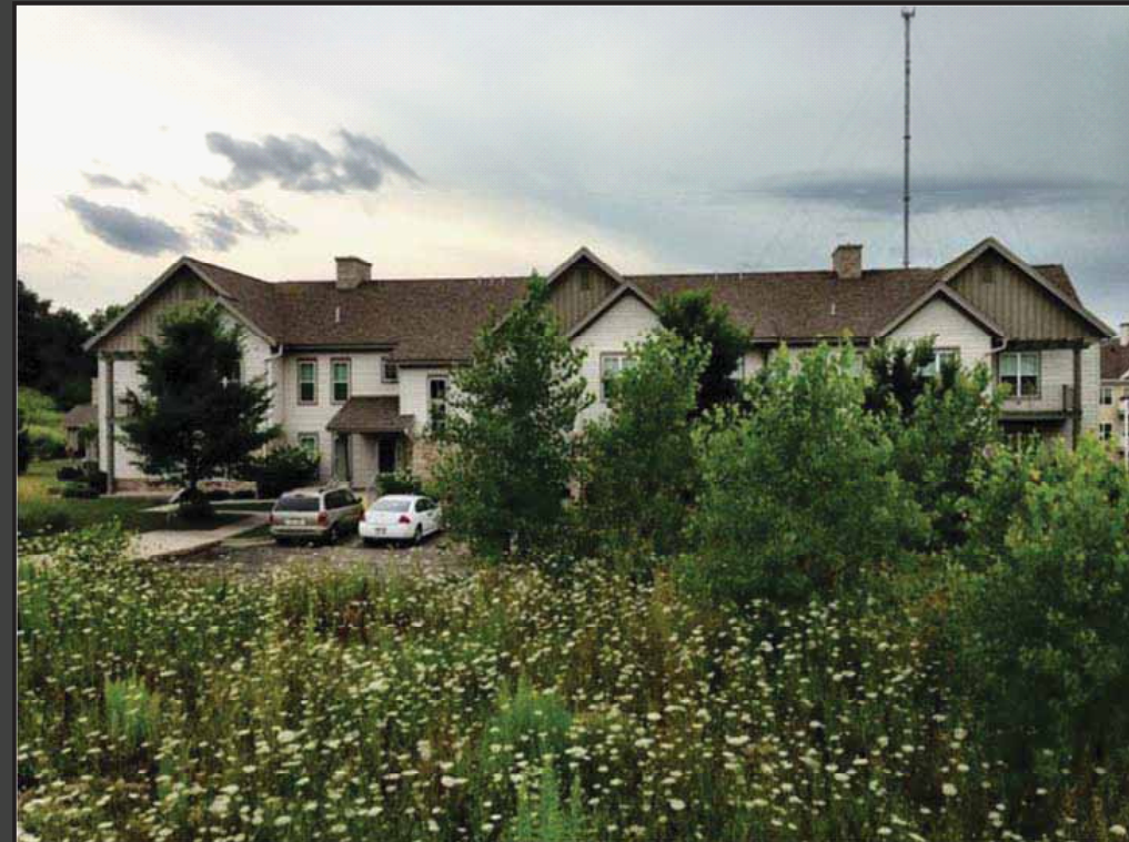
12 UNIT CONDEO, HILLSIDE ESTATES
