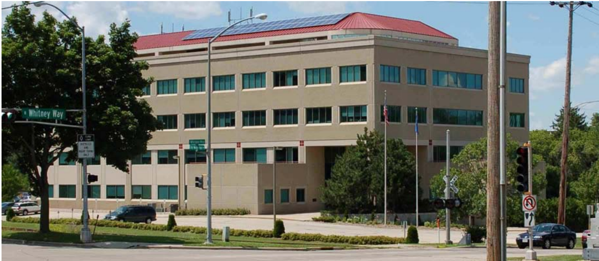
610 N. Whitney Way, "PSC Building"
