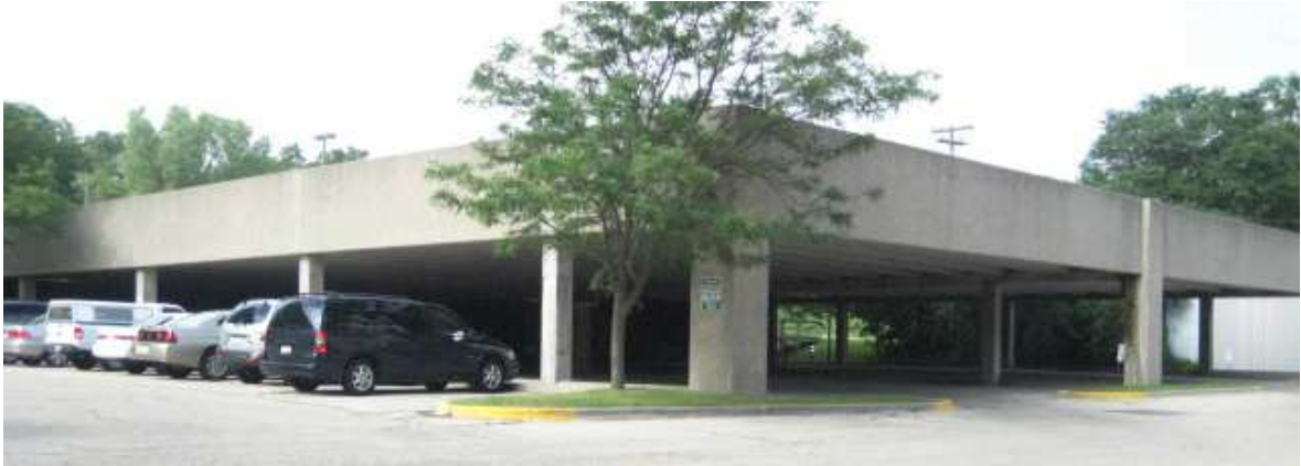
610 N. Whitney Way, "PSC Parking Ramp"
