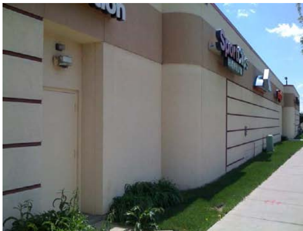
Figure 3c: Back of retail building facing Gammon Road.
