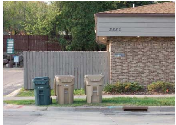
Figure 3b: Back of a retail building facing University Ave.
