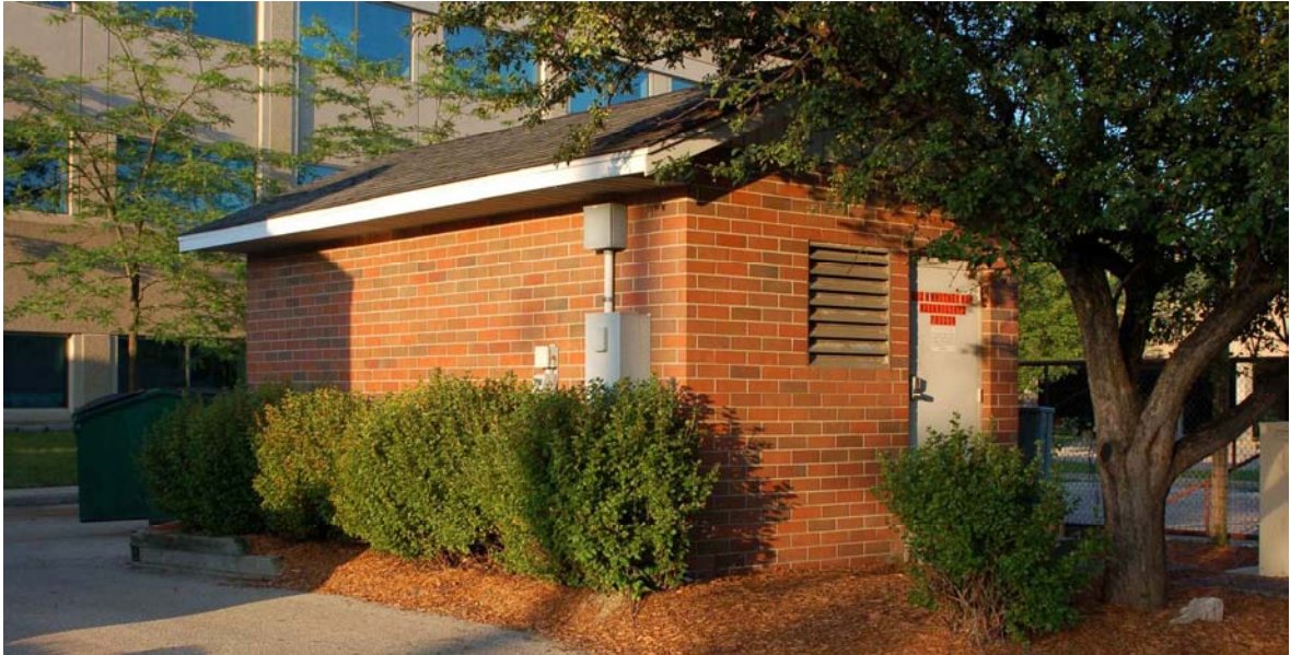
Easement, "AT+T Utility Shed"
