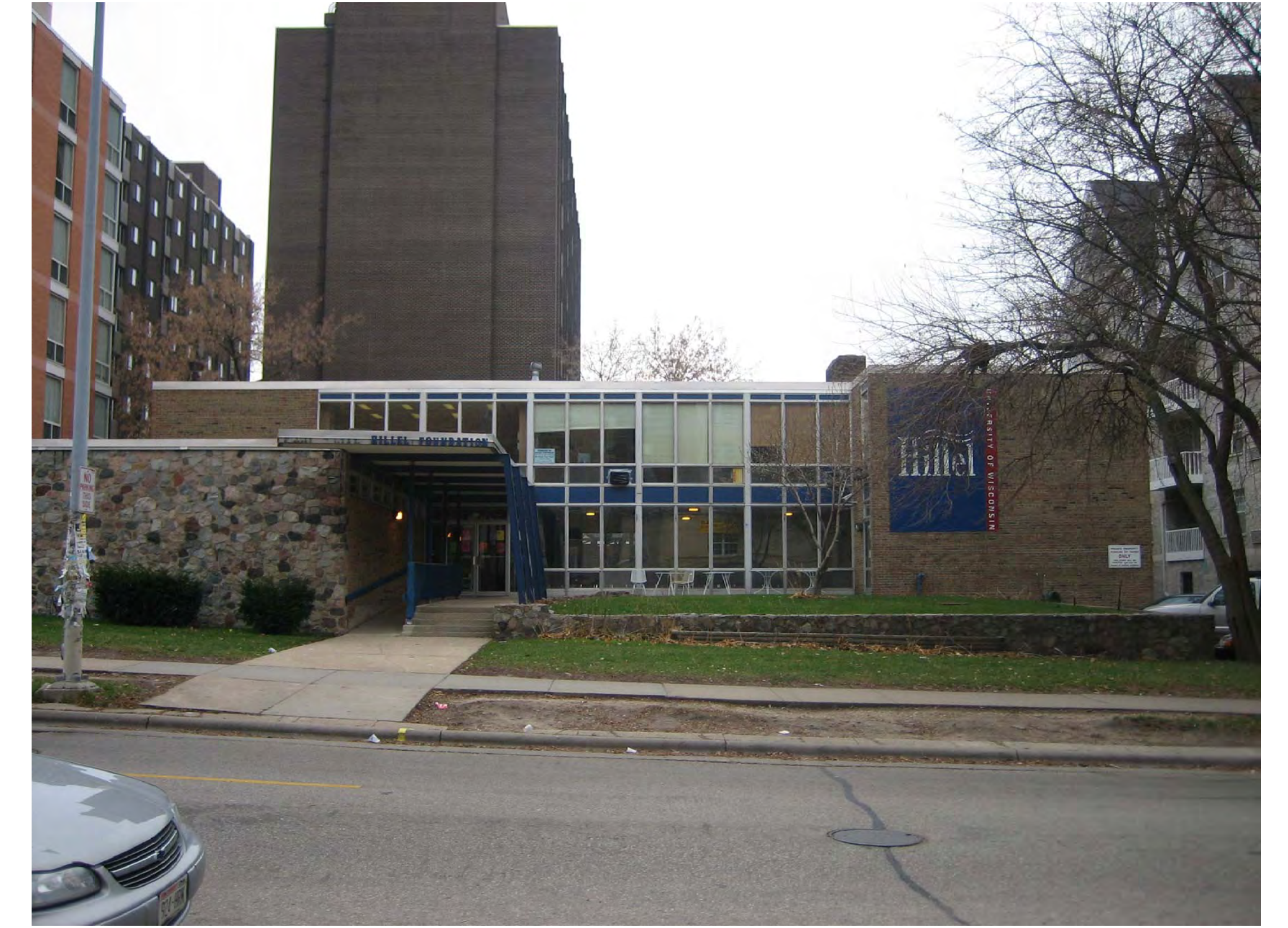
PHOTO 3 View looking south across Langdon Street (Existing Hillel building)
