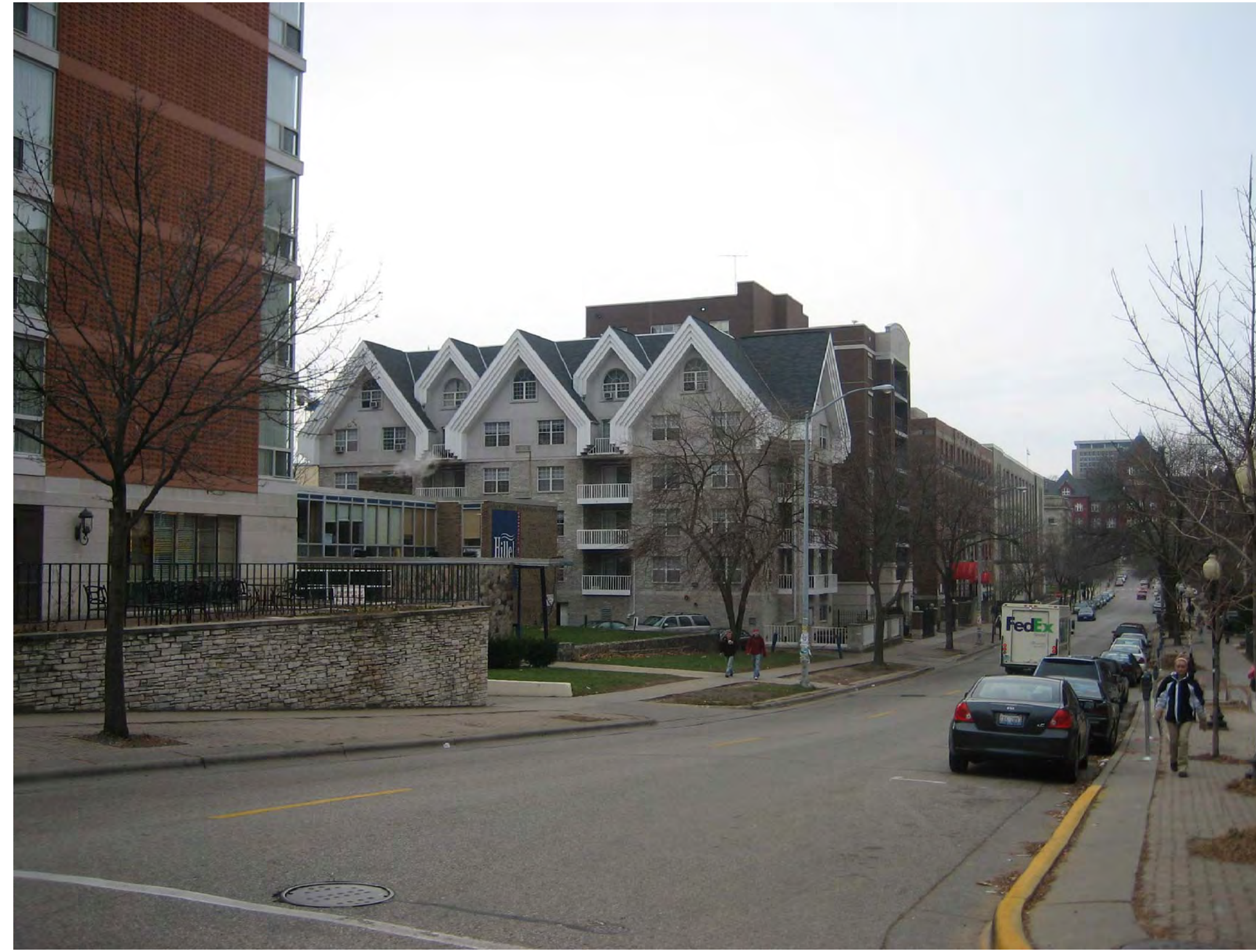
PHOTO 2 View looking southwest to Hotel, Hillel & Residential Buildings
