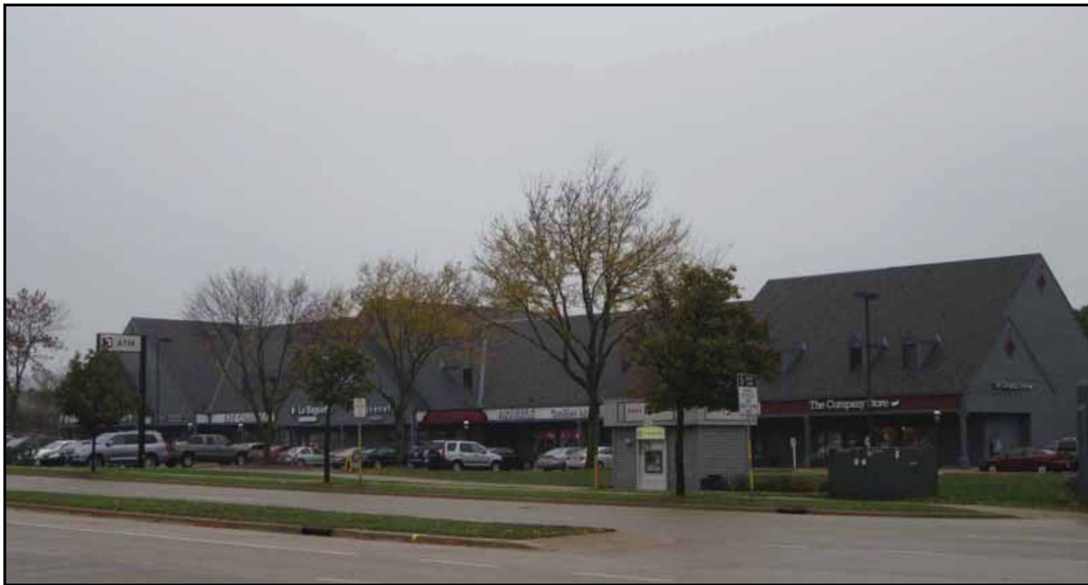
Adjacent Property to Northwest
