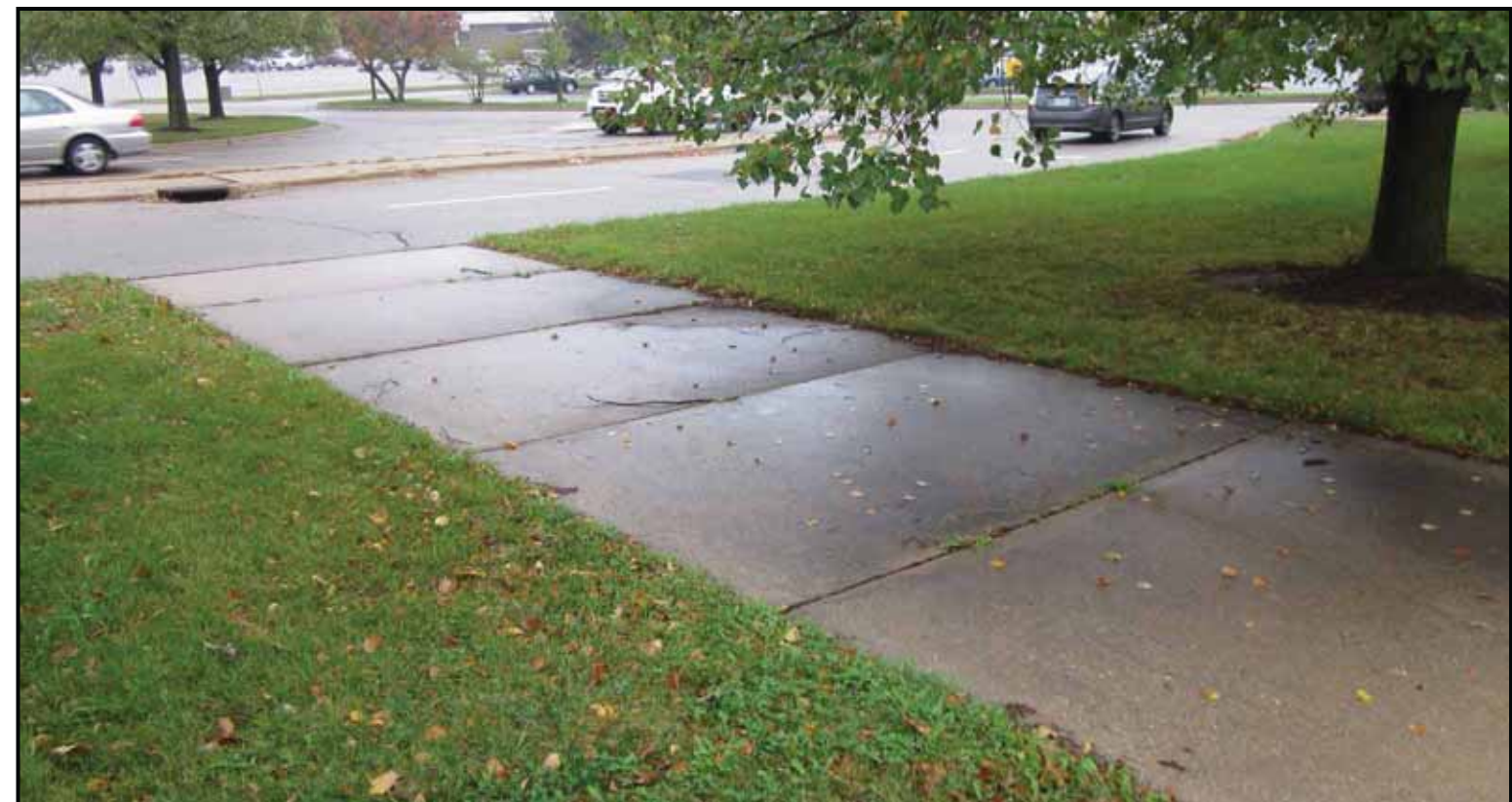
Sidewalk Connection to S. Westfield Road Entrance to West Towne Mall Development
