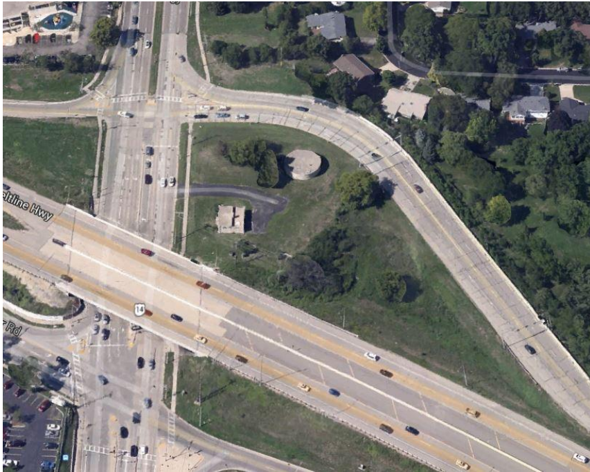
An aerial view showing the pump house and the reservoir along South Whitney Way. The reservoir is the round building to the north of the pump house.
