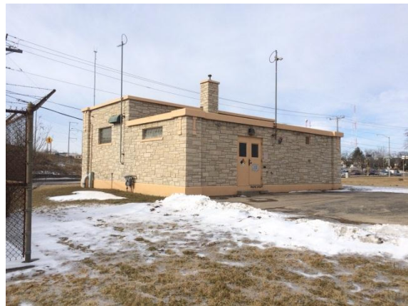
The rear of the building where the addition will be located
