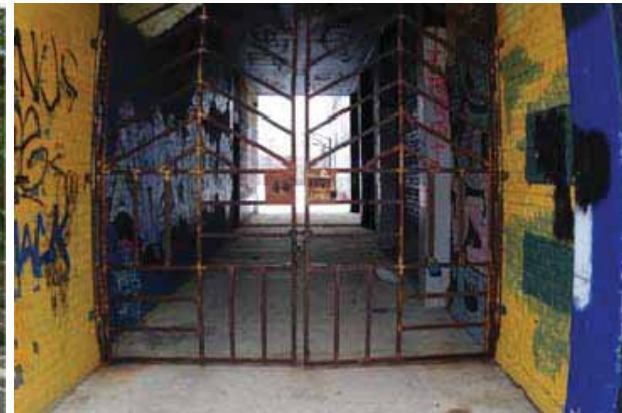
2 VIEW OF TUNNEL FROM E. WASHINGTON AVE. SIDEWALK
