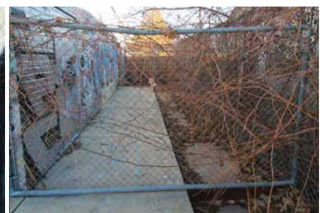
7 VIEW BEHIND EXISTING BUILDING
