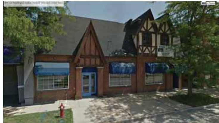
1 VIEW OF FACADE ALONG EAST WASHINGTON
