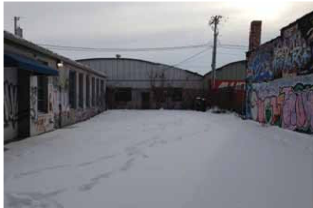
4 VIEW SOUTHEAST INSIDE COURTYARD
