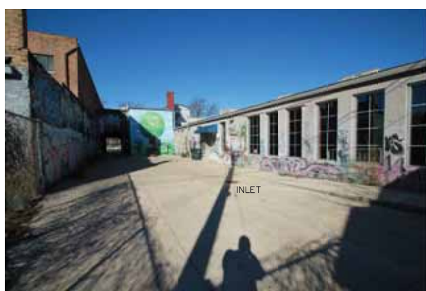
8 VIEW NORTH INSIDE COURTYARD
