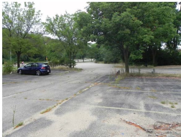
9 VIEW TOWARDS JOHN NOLEN DRIVE LEAVING THE SITE
