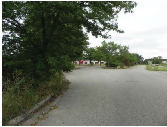
1 ENTERING SITE FROM THE JOHN NOLEN DRIVE ACCESS ROAD
