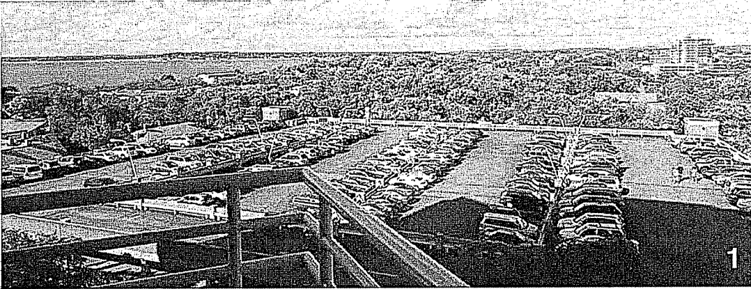
4:42 pm Capitol North Ramp full. A waiting car cannot enter ramp until one leaves, backing up Mifflin traffic onto Webster.
