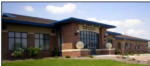
West District Station
