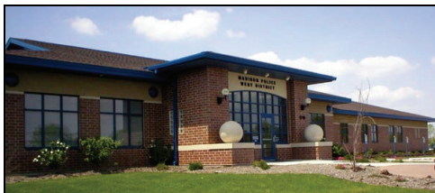
West District Station
