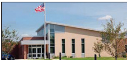
East District Station
