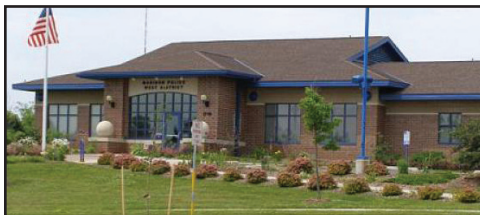
West District Station
