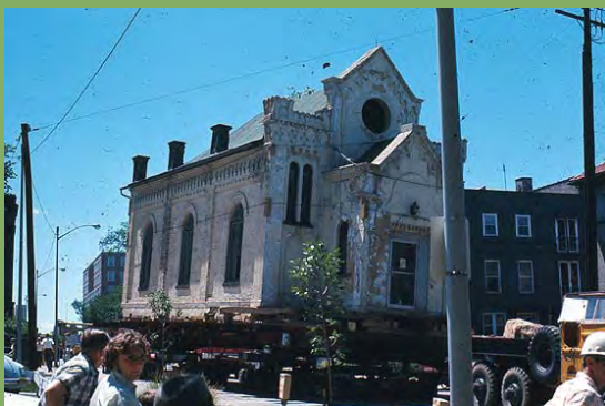
Photo: Transporting the building from 214 West Washington to 302 East Gorham Street (James Madison Park).
