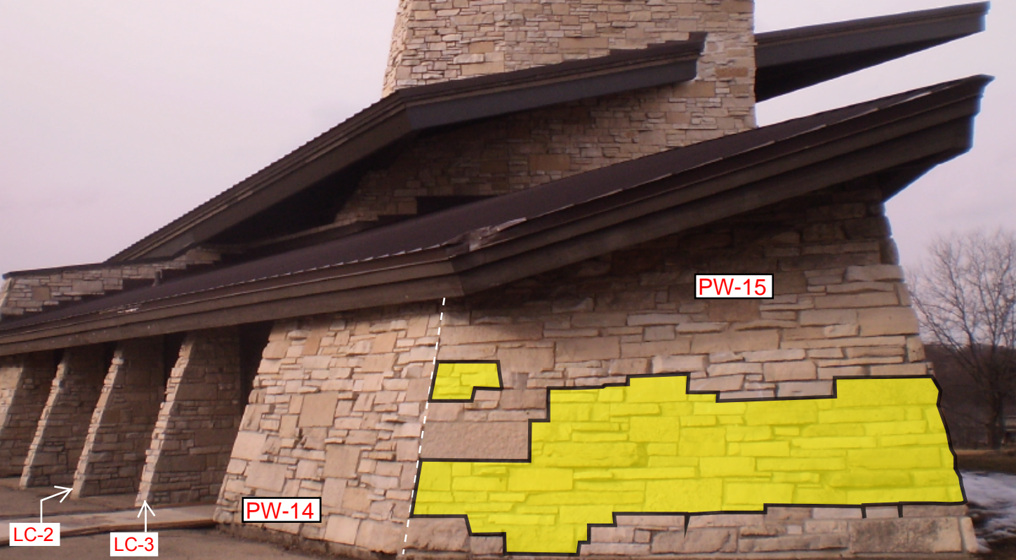
Instructions- Repoint joint shown in shaded areas on wall PW-15
