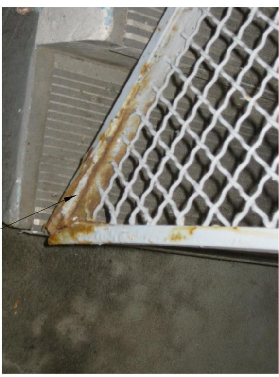
CLEAN MESH GUARDRAIL TO WHITE METAL APPEARANCE AND PAINT. PAINT COLOR TO BE SILVER, SEE SPECIFICATIONS
