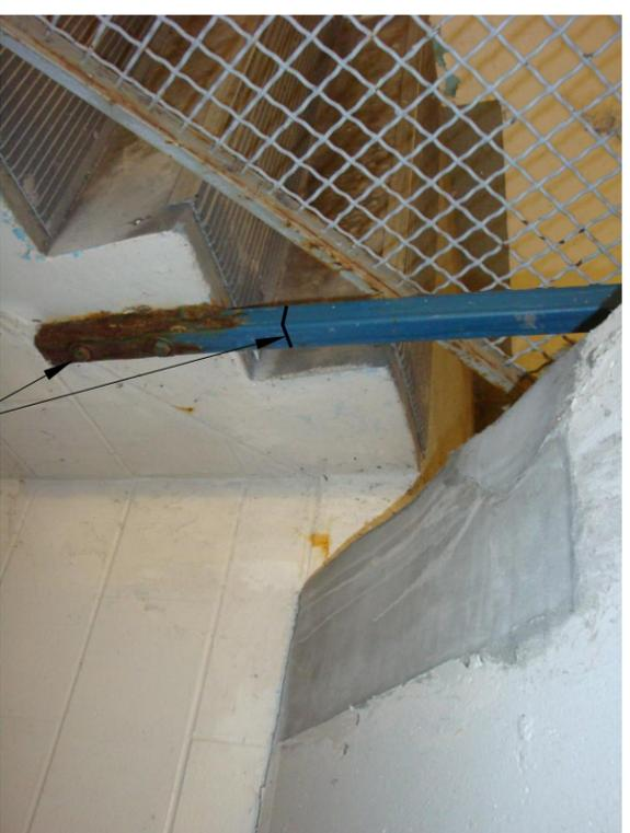
CUT OFF BOTTOM OF GUARDRAIL SUPPORT POST, WELD NEW SECTION TO POST TO REMAIN AND RE-ANCHOR TO STAIR RISER, BID ITEM #23
