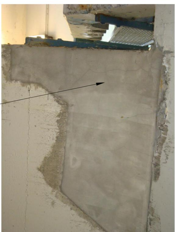
CONCRETE RESTORATION AT UNDERSIDE OF STAIR, BID ITEM #5
