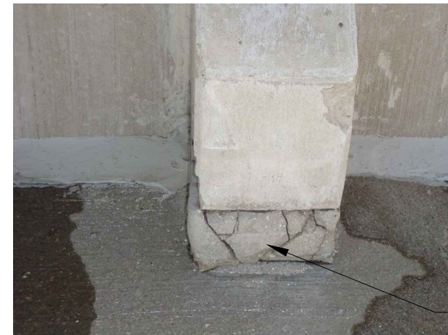
6 PHOTO OF CRACKED HAUNCH GROUT D2 SCALE : NTS
