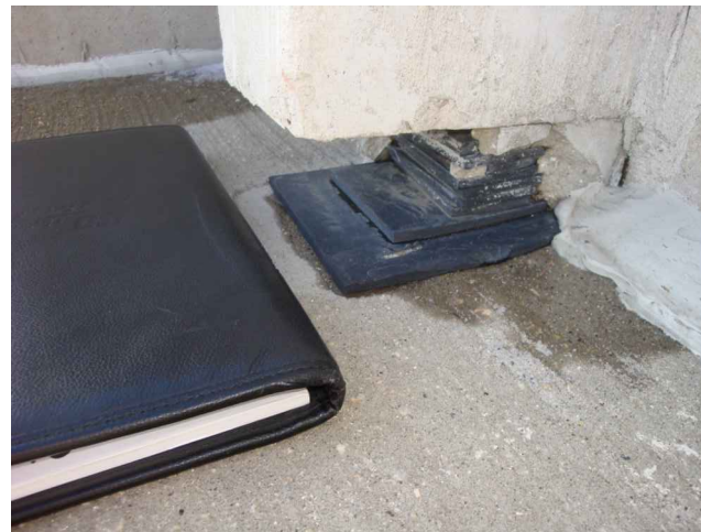
5 PHOTO OF HAUNCH PLATE STACK D2 SCALE : NTS
